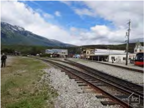
Railroad right of way located north of the subject parcel. Note that there are two small lots located between the subject parcel and the railroad right of way
