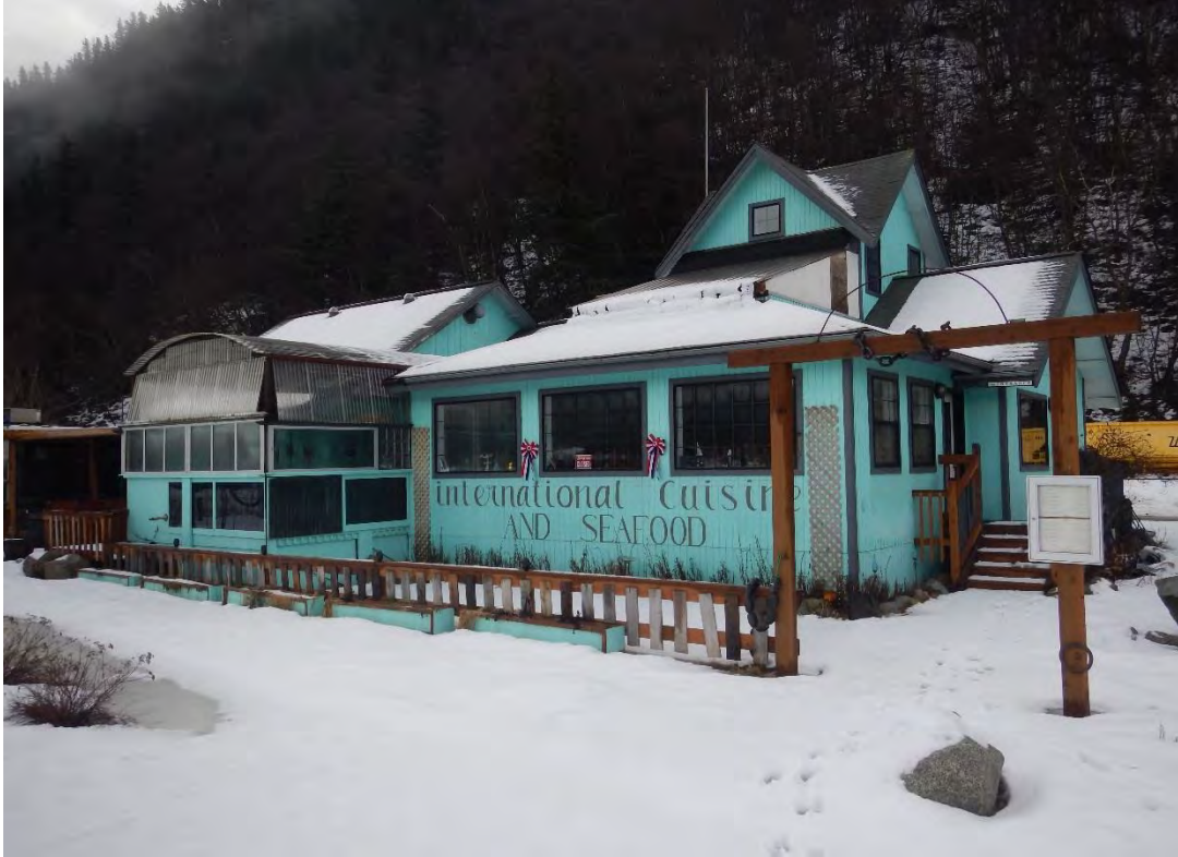
PHOTO 1 – Looking NE onto subject property from sea walk. (031418_1744)
