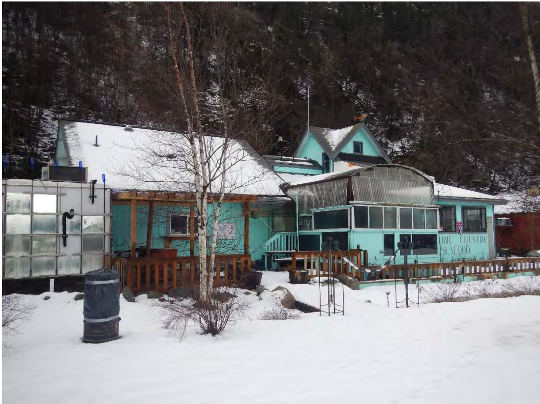
PHOTO 2 – Looking approximately SE across property from sea walk. (031418_1745)
