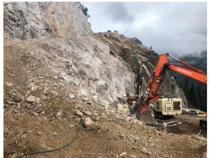
Installation of rock anchors during construction of Wall 15A on White Pass & Yukon Route Railway.
