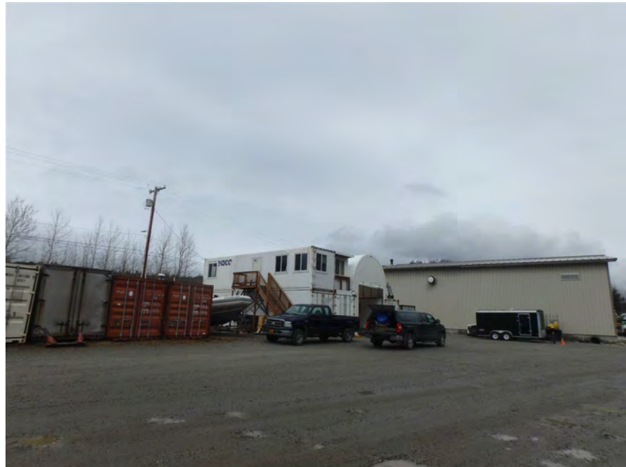
Looking northwest at subject, which begins to right of the red boxes
