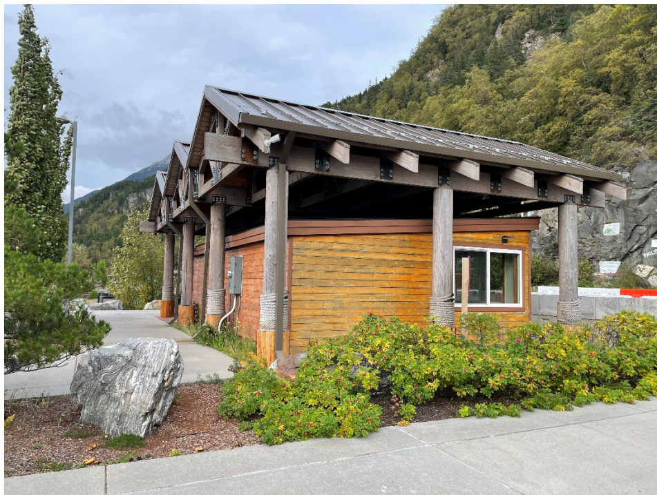
PHOTO 2 – Subject exterior looking in a northerly direction. (091922 (570))
