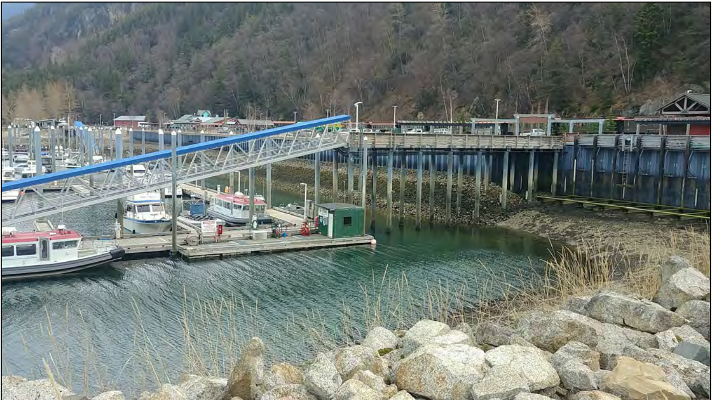
Photograph 6. View of floating fuel dock.
