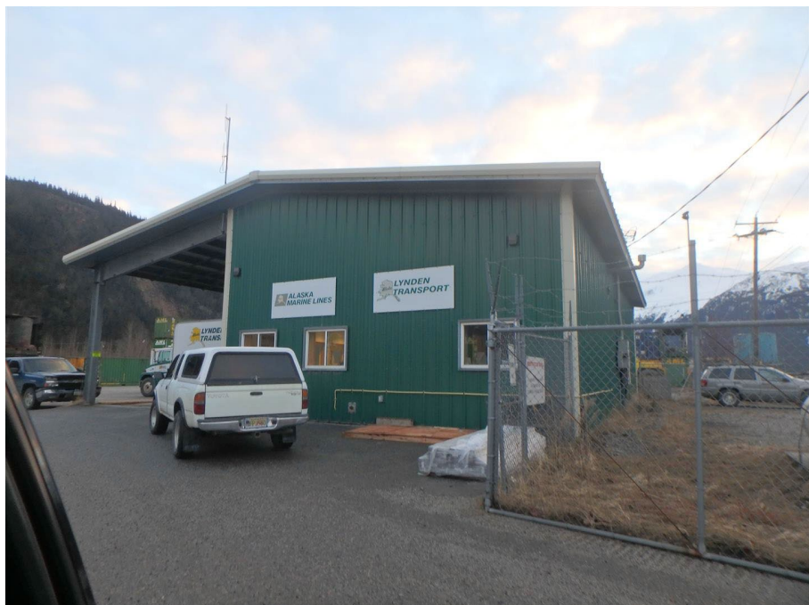
North end of subject building
