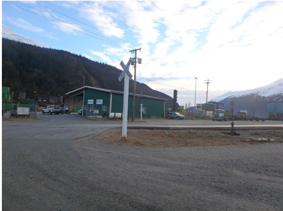
View of subject from northwest
