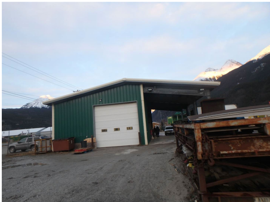
South end of subject building
