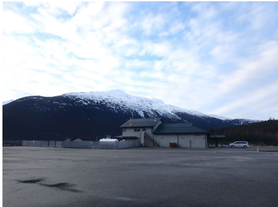
Looking northeast at subject across Ore Dock loading area, from near the dock itself
