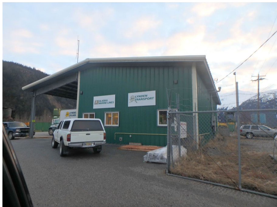
North end of subject building
