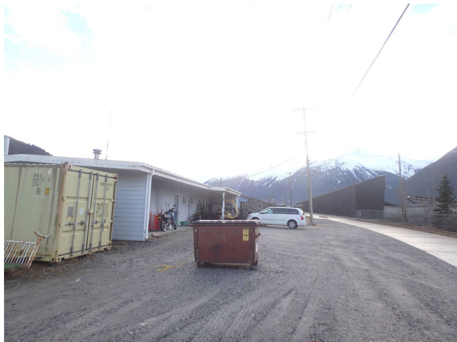
West side of subject building, road continues to ore terminal
