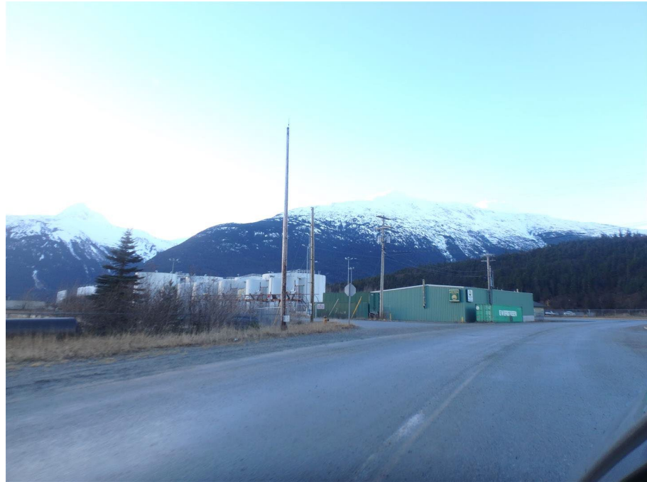
View of Subject approaching from east along Terminal Way
