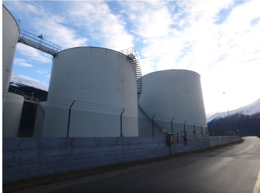
South end of tank farm
