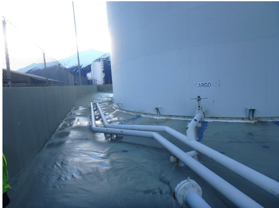
Looking west along south end of containment area, tank 14
