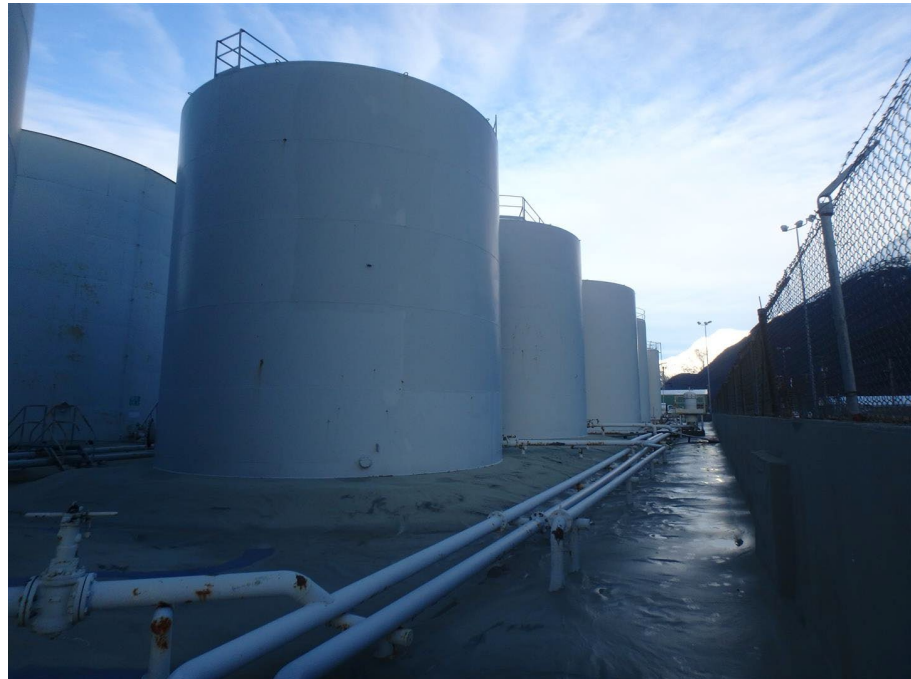
Looking northeast from southeast corner of containment area, tank 13 at center
