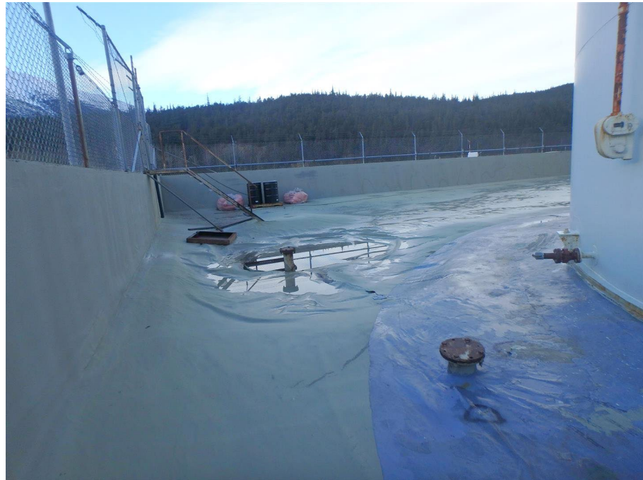
Fence, wall, pump and membrane detail southwest of tank 14
