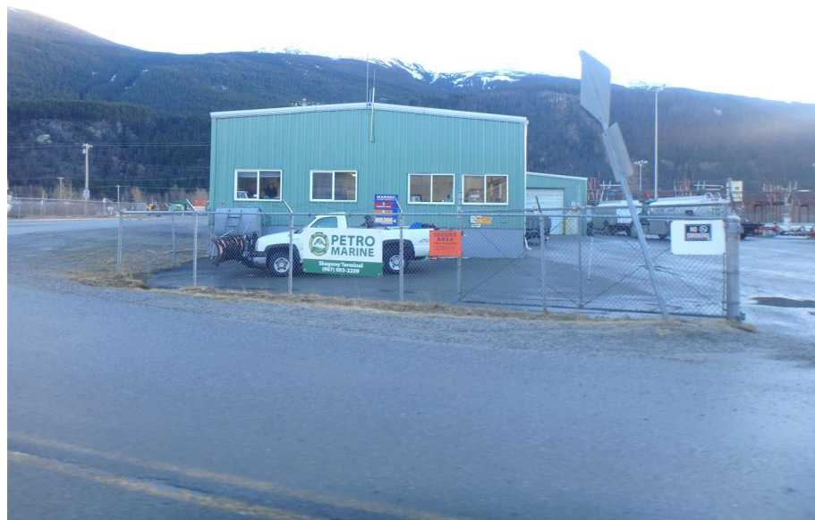
Warehouse/office from west
