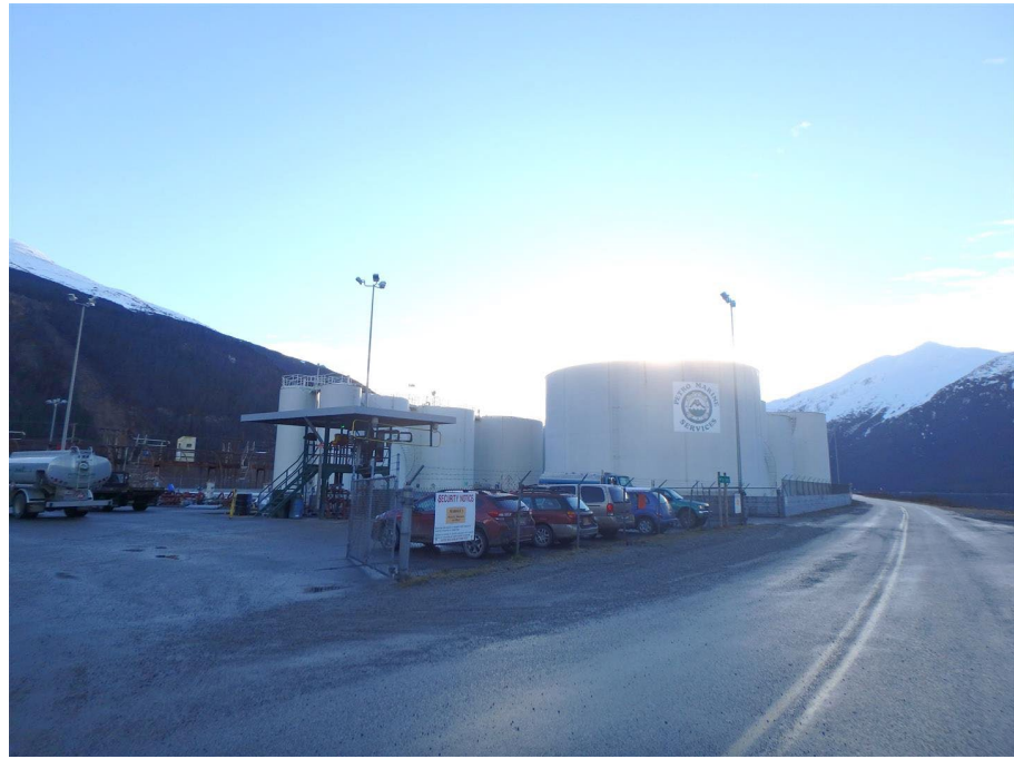
Gated entry and tank farm from north
