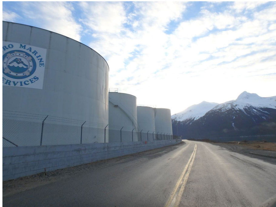
Middle of tank farm along Terminal Way
