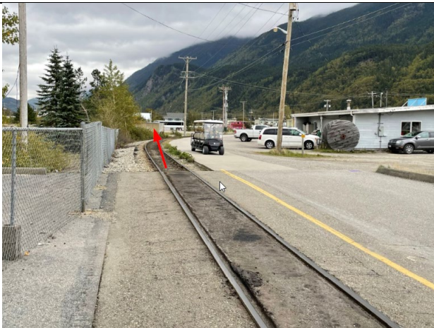
Looking NE from the end of pavement toward track realignment extending toward Terminal Way.
