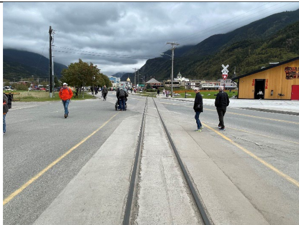
SW end of segment 4 looking NE across Broadway right-of-way. Note this segment appears to be mostly concurrent with existing highway ROW.
