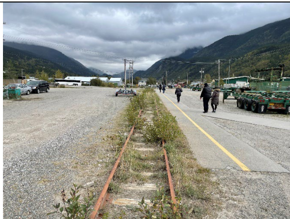
Mid to SE section of easement looking NE.
