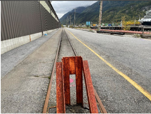
SW end of easement looking NE. The first ~ 700 feet has railroad track.
