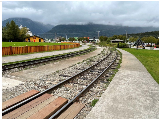
Looking west from the eastern end of segment 6. Crossing in photo foreground not on site.
