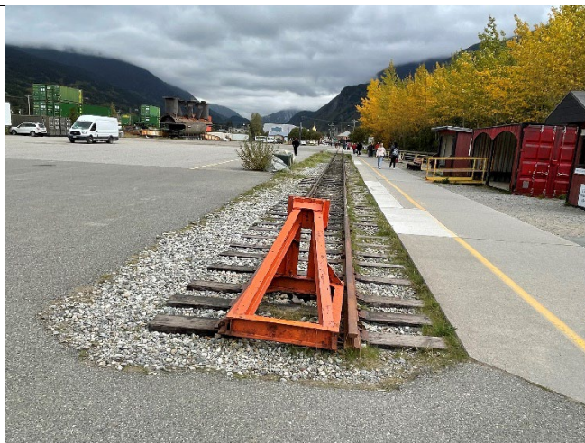
SW end of segment 3 looking NE.
