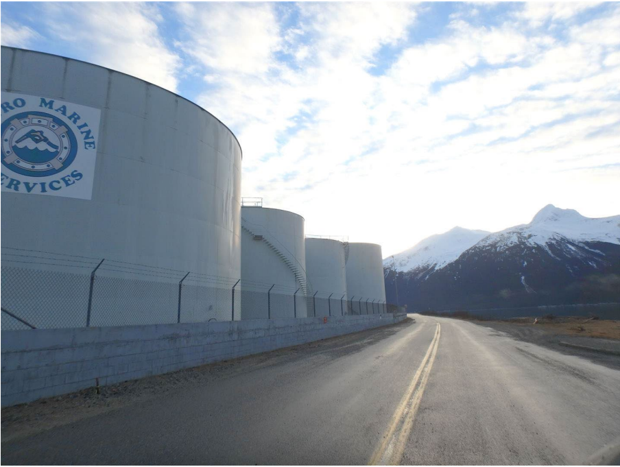
Middle of tank farm along Terminal Way
