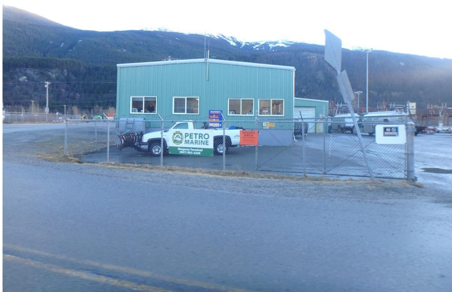
Warehouse/office from west
