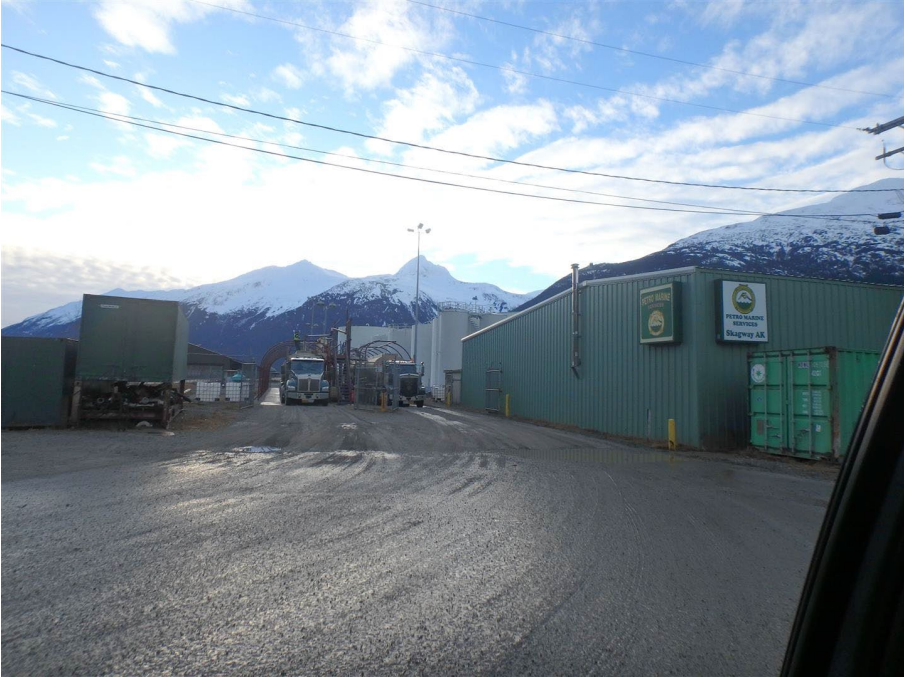
Bonded double TTLR along west side of subject
