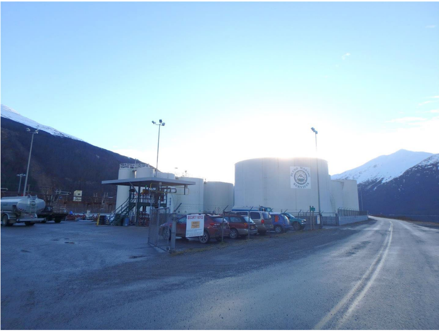
Gated entry and tank farm from north
