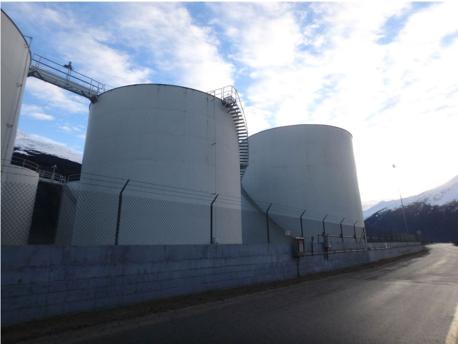
South end of tank farm
