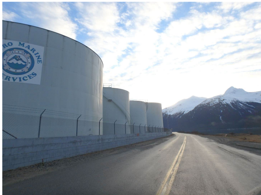
Middle of tank farm along Terminal Way
