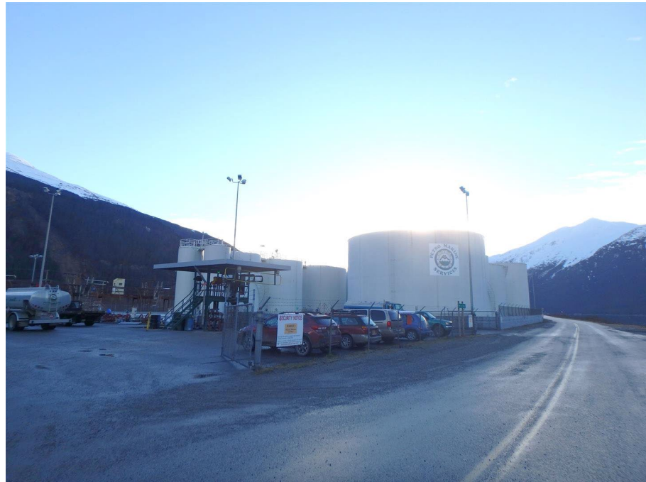
Gated entry and tank farm from north
