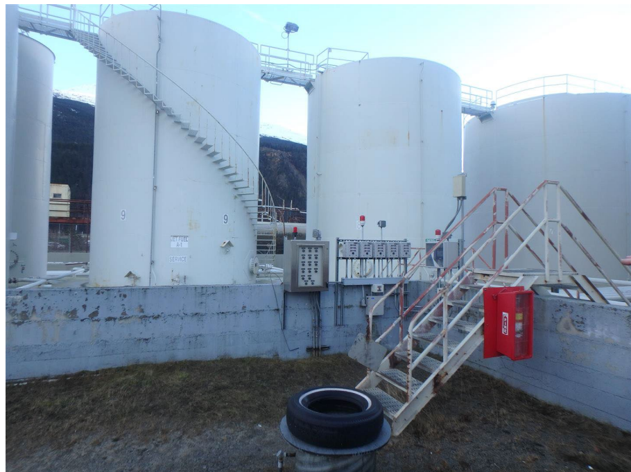
Alarm area outside containment wall perimeter, north end
