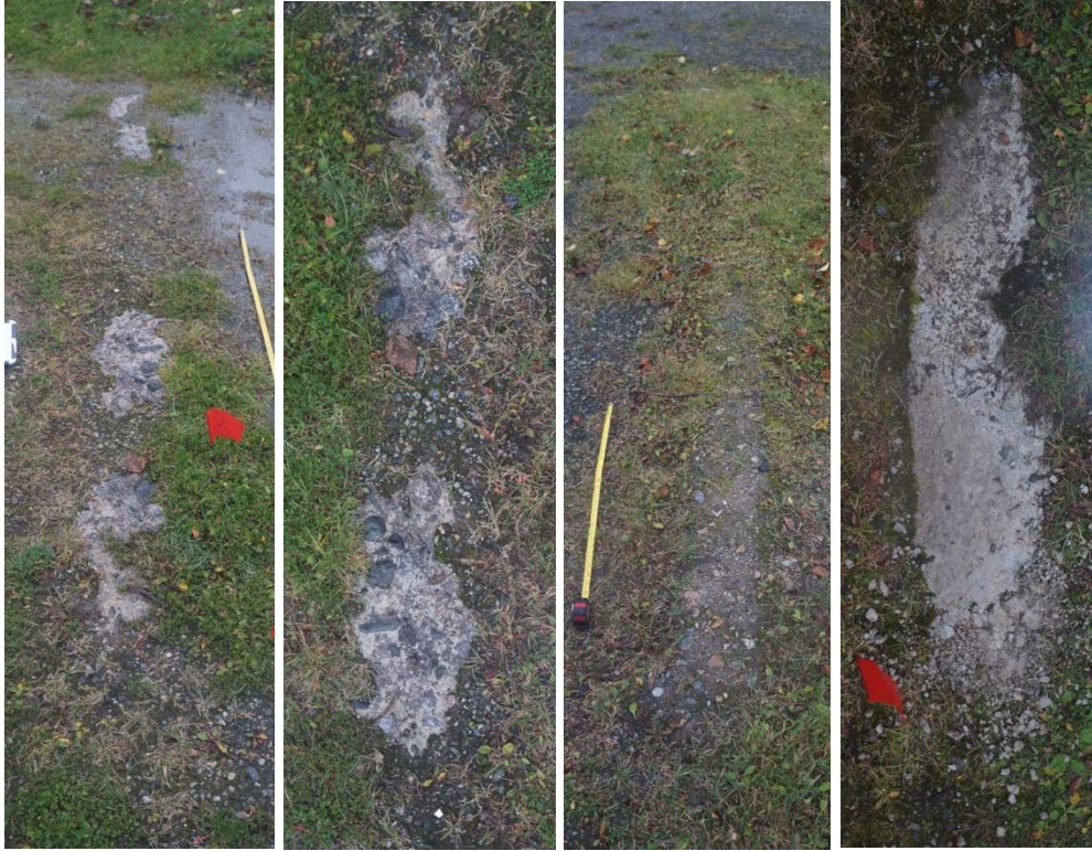
Figure 20. In-situ foundation elements. (a) Foundation (320 x 25 cm, oriented NW-SE) of eastern wall. (b) Close-up of the cement fill. (c) Buried foundation (320 x 25 cm, oriented NW-SE) of western wall. (d) Coated foundation element near northern wall (110 x 25 cm, oriented SW-NE).
