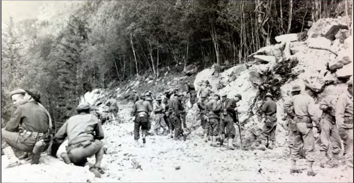
Building West Creek Road, Photo courtesy of Andrew Beierly
