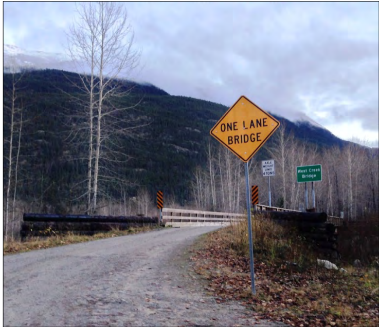
West Creek Bridge
