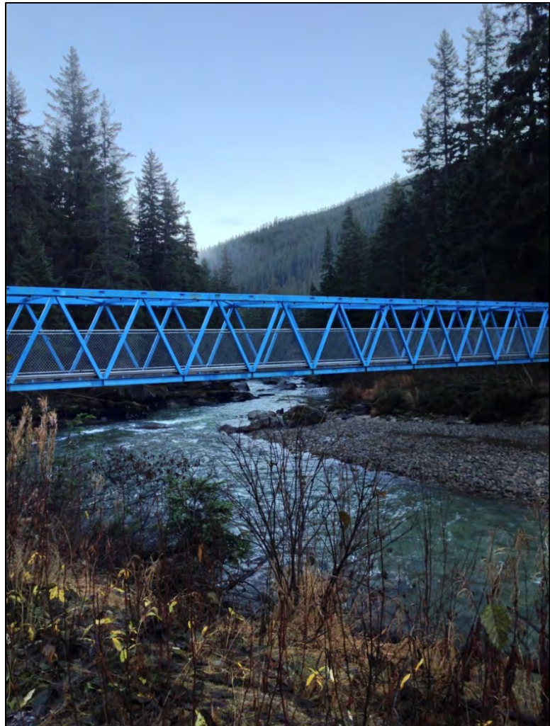
Jay Frey Recreation Bridge
