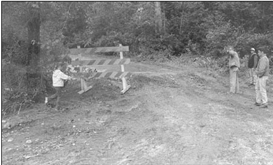
Wayne Ames shows his wife Shannon and friends how the creek cut through the old Hanousek property and came down the road just before the West Creek Bridge. City workers were able to put part of the road back together to allow access for raft tours on the nearby Taiya River. Jeff Brady, Skagway News
