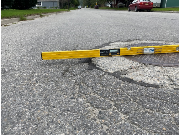
Photo 7 Example of manhole lid above grade
