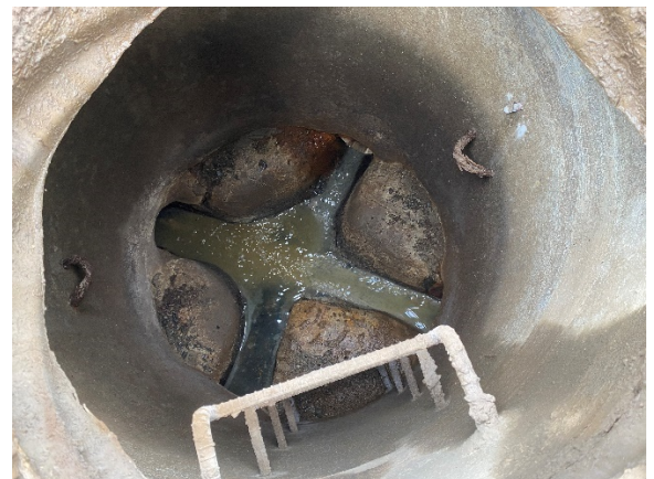
Photo 24 Example of a sanitary sewer manhole
