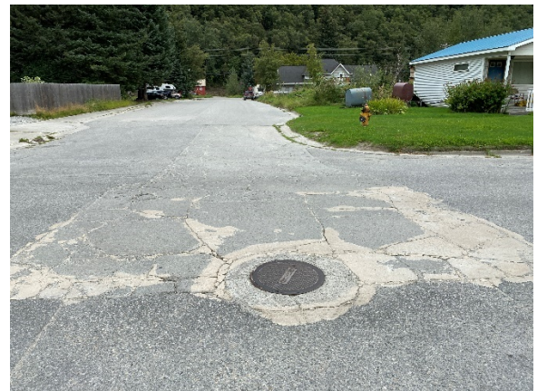
Photo 18 Example of concrete patch
