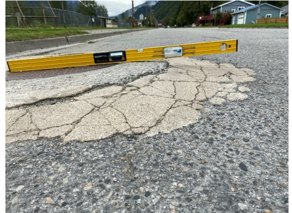
Photo 8 Example of manhole lid above grade
