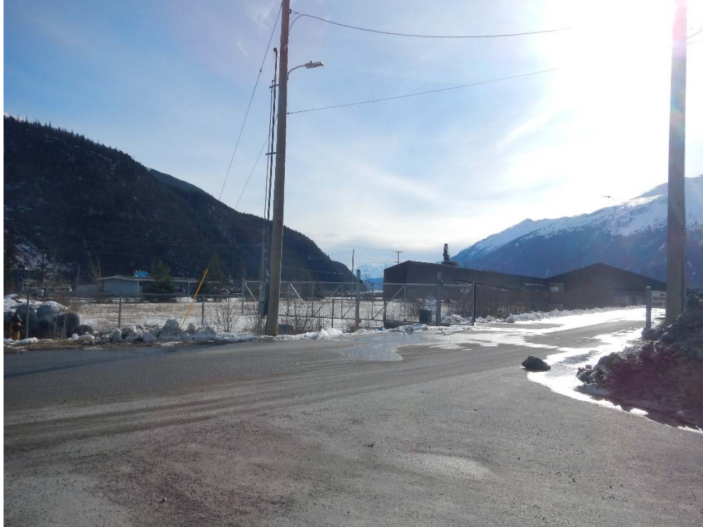
PHOTO 3 – TL 6A LOOKING SOUTHEAST FROM ENTRANCE TO ORE TERMINAL. (031418_1806).
