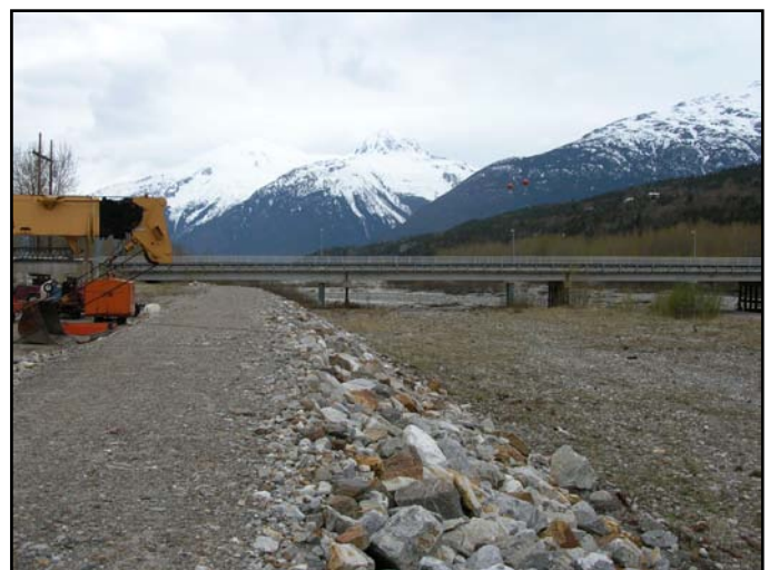
Skagway River Dike, May 2008
