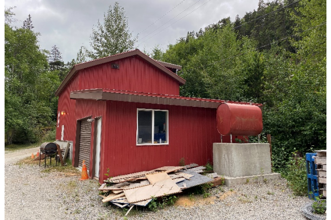
Figure 104: Training Windows in Hose Tower at Fire Hall
