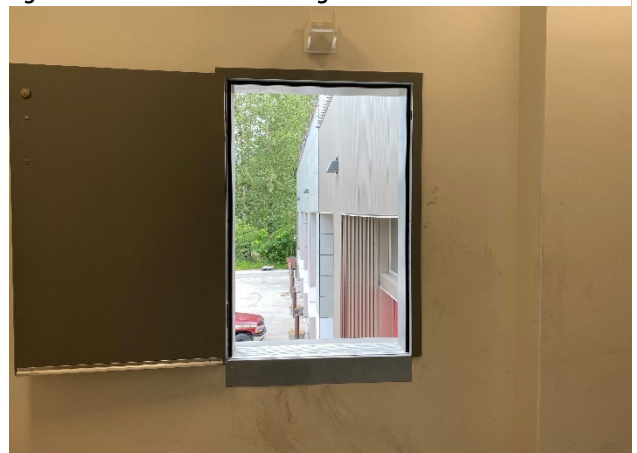
Figure 107: Hose Tower Training Window
