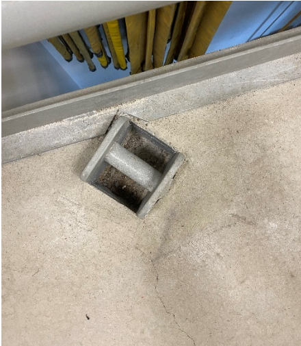
Figure 108: Rope Rescue Anchor Points - Fire Hall Hose Tower
