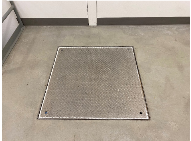
Figure 109: Confined Space Lifting Point - Fire Hall Hose Tower
