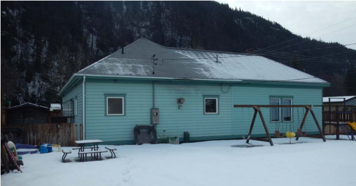
PHOTO 2 – WESTERN SIDE OF THE SUBJECT BUILDING FROM THE FENCED IN YARD. (031418_1761)
