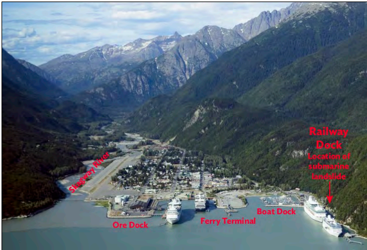
Figure 5-10: The Location of the 1994 Submarine Landslide
