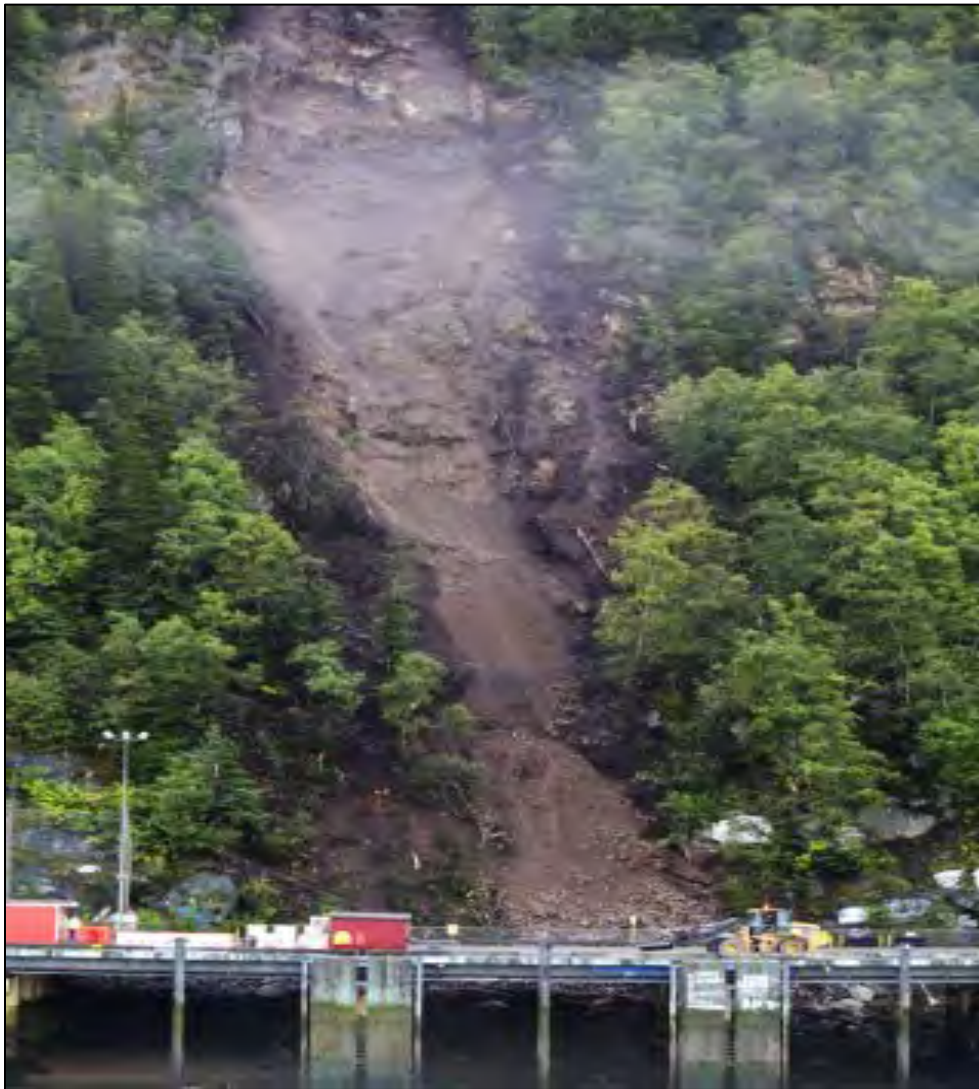
Figure 5-6: Site of Rockslide in Skagway, Alaska
