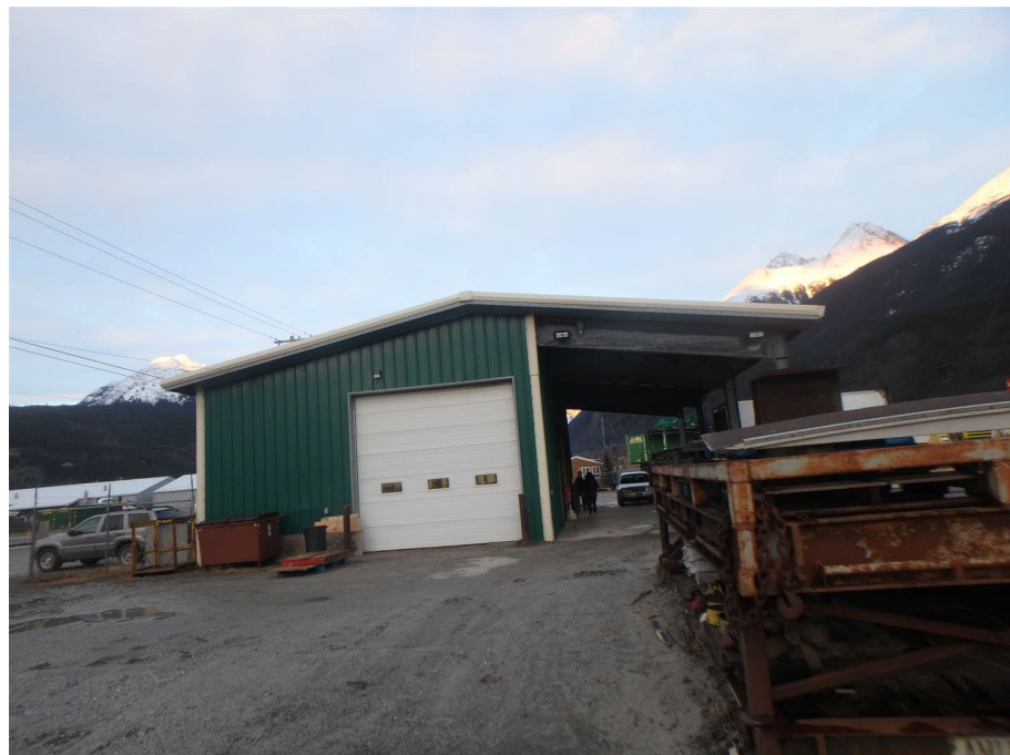
South end of subject building
