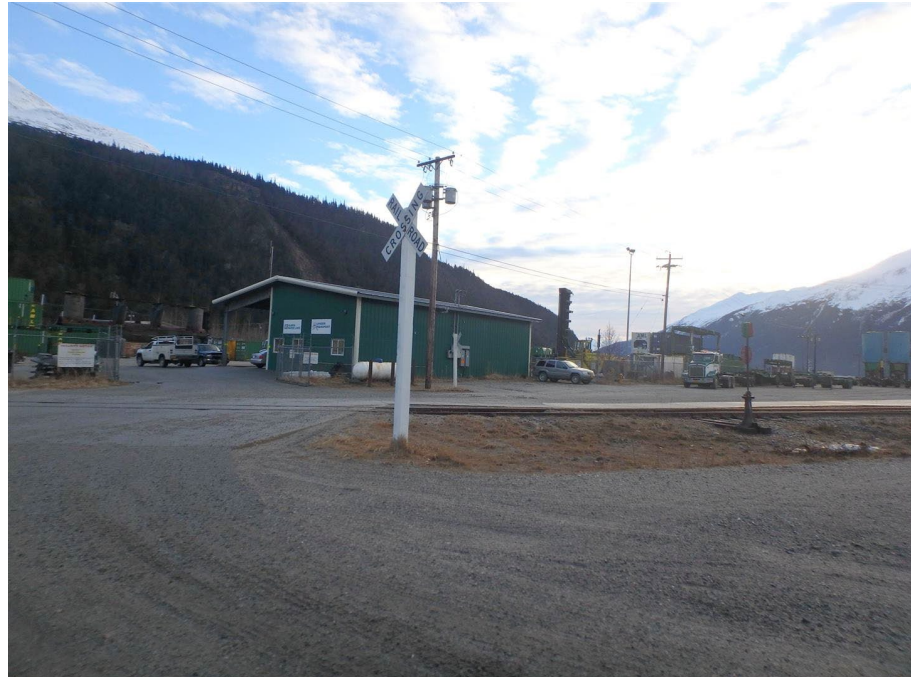
View of subject from northwest
