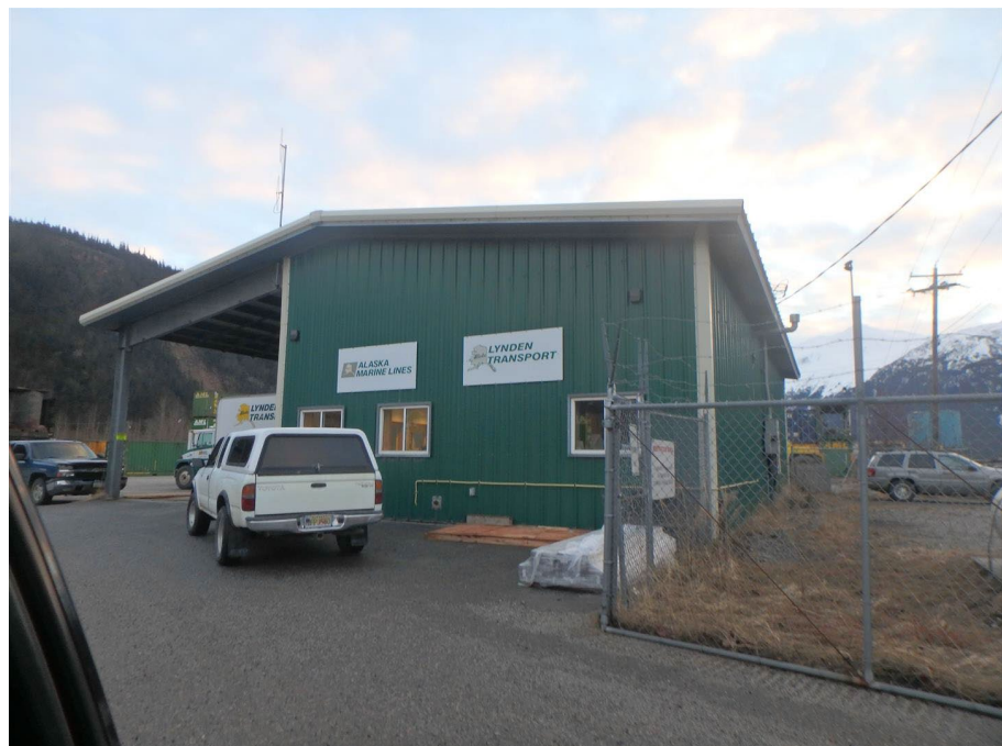
North end of subject building
