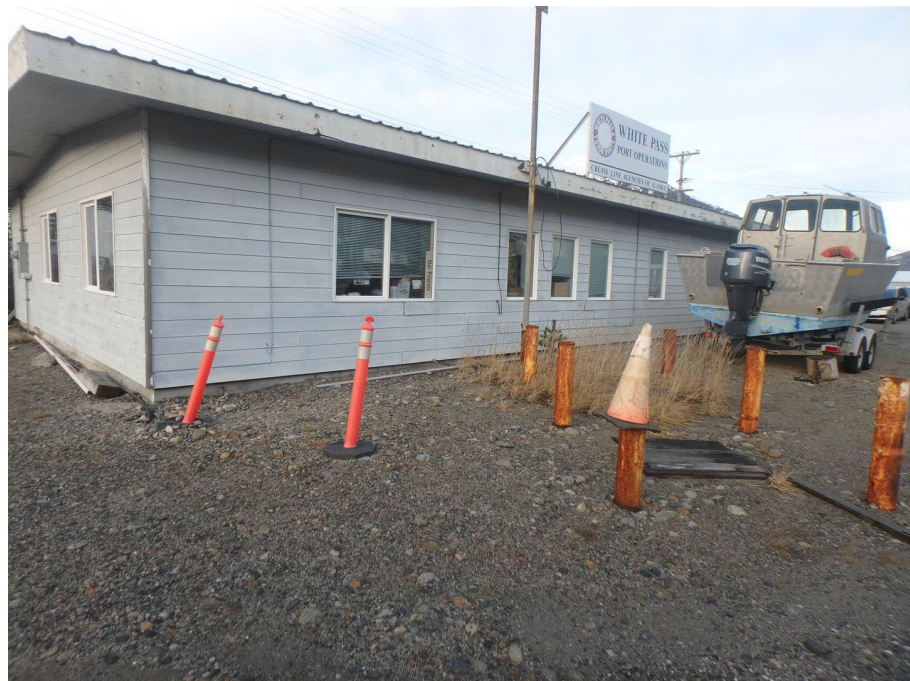
East side of subject building
