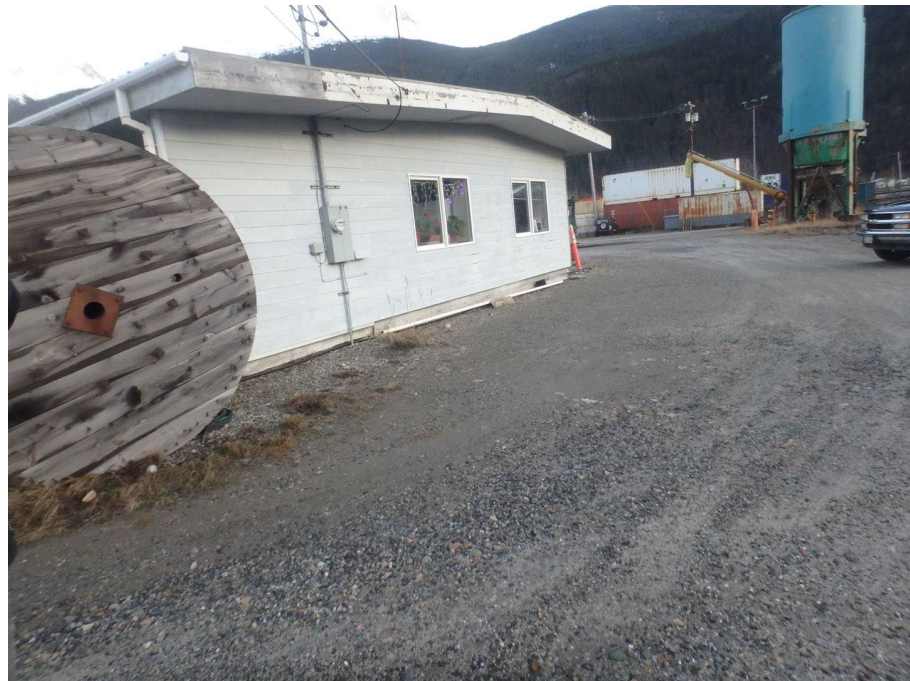
South side of subject building facing east
