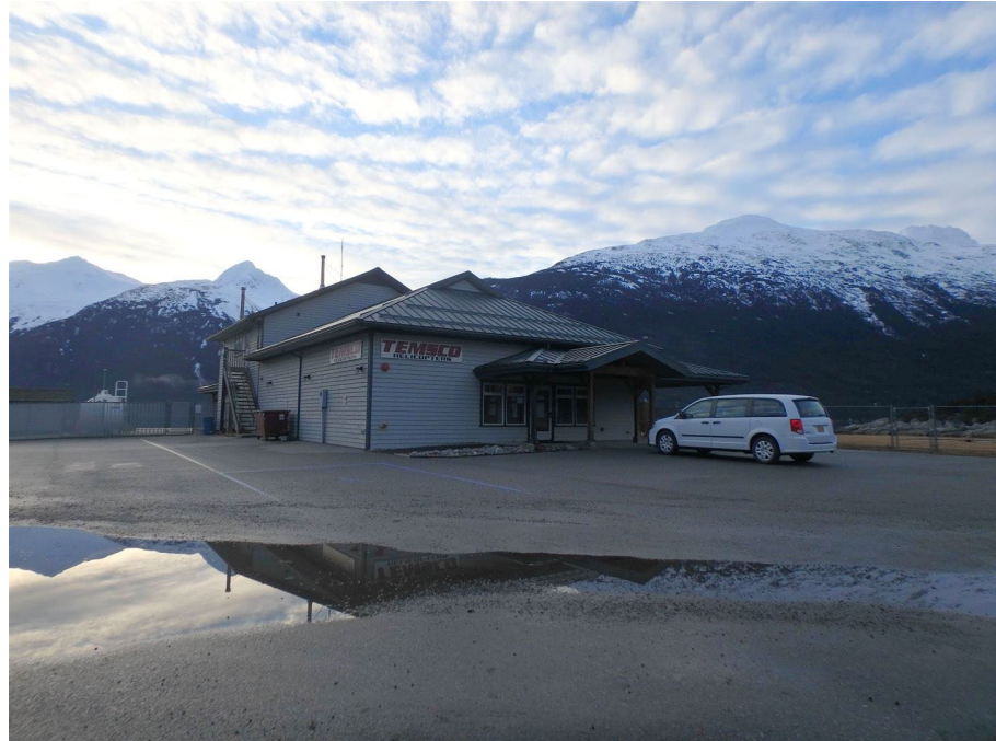
View west at subject from approximate premises corner
