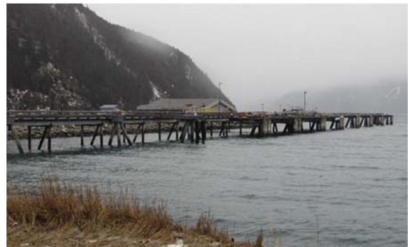
Broadway Dock with AMHS Terminal in Background
