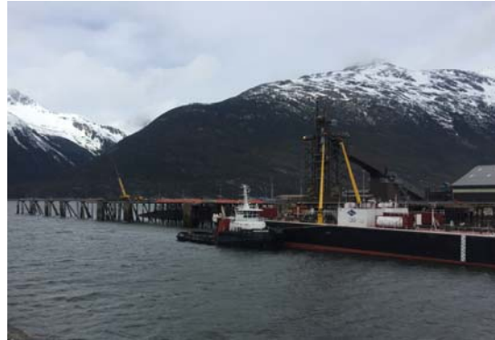
Ore Dock at Skagway Ore Terminal and Shiploader
