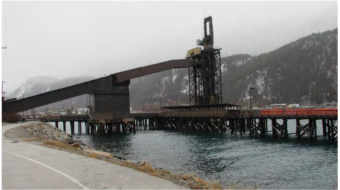
FIGURE 2-1. SKAGWAY ORE DOCK AND SHIPLOADER
