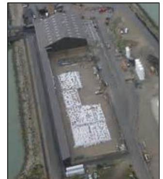
concrete pad staging area
