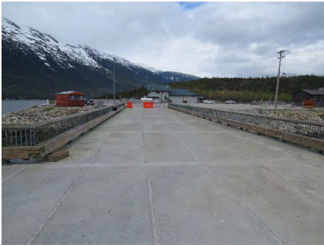
Photo 42- Concrete approach to concrete platform
