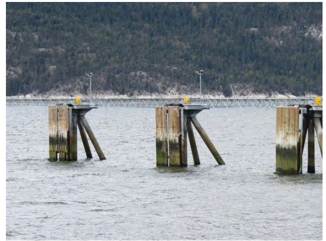
Photo 2- Dolphin addition (1 of 2)
