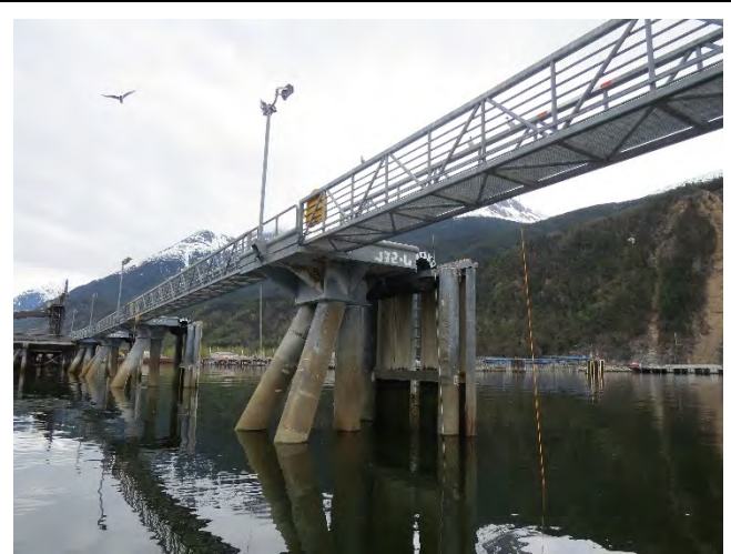
Photo 50- Dolphin addition (4 of 6)
