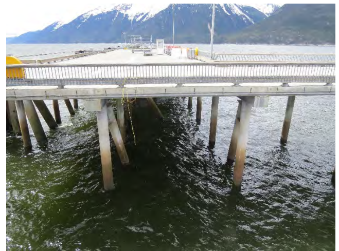
Photo 39- Concrete platform (2 of 4)
