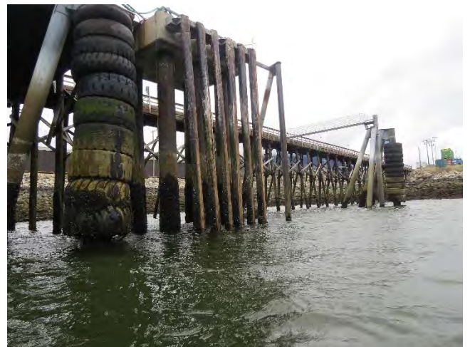
Photo 18- North timber platform, near AML3 and DI (2 of 4)
