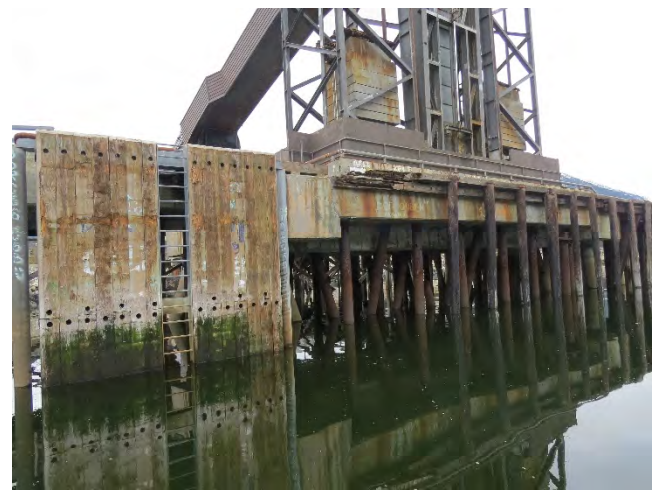
Photo 8- Ore ship loader platform (1 of 3)
