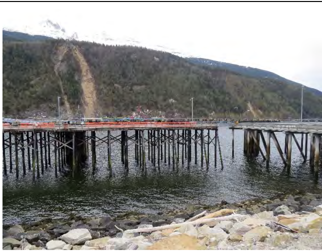
Photo 36- South timber platform, (2 of 3)
