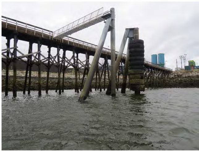
Photo 19- North timber platform (3 of 4)
