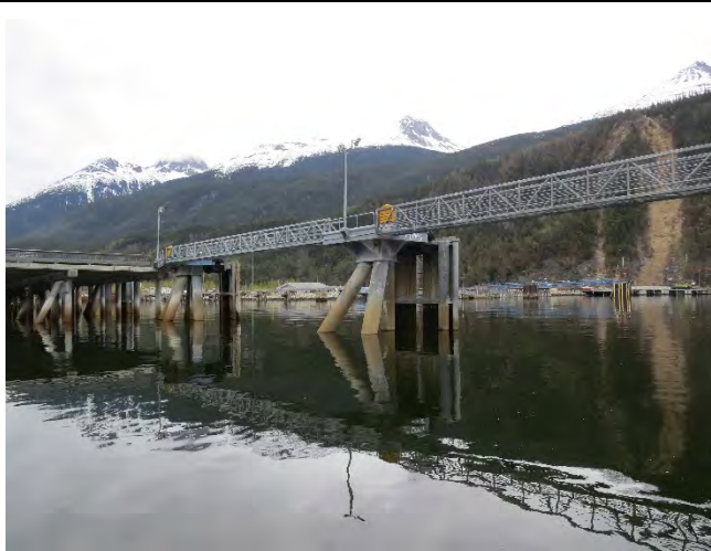
Photo 49- Dolphin addition (3 of 6)
