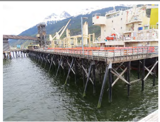
Photo 37- South timber platform, (3 of 3)
