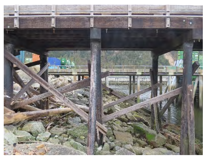
Photo 22- North timber platform (2 of 7)
