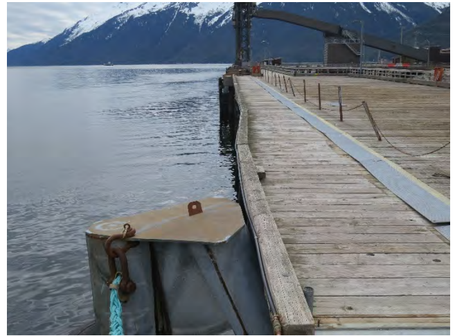
Photo 89- Old portion of dock
