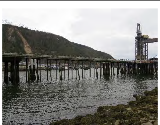
Photo 27- North timber platform (6 of 7)
