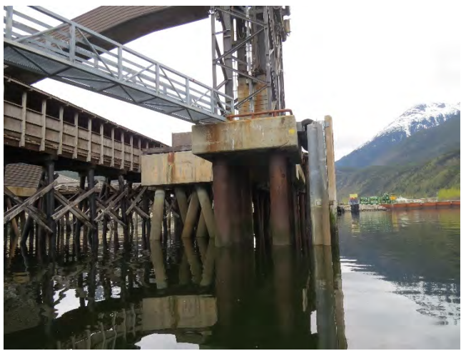
Photo 7- Ore ship loader dolphin, painted steel with concrete cap
