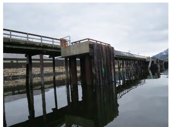
Photo 12- - Ore ship loader dolphin, steel with concrete cap
