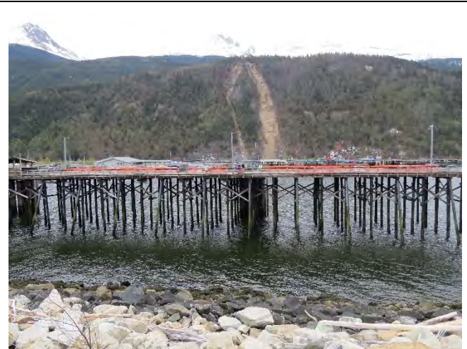
Photo 35- South timber platform (1 of 3)
