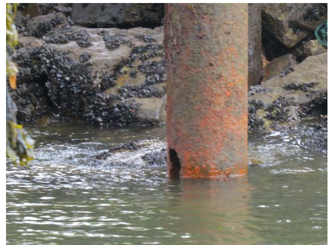
Photo 85 - Enlargement of steel pile (previous image)
