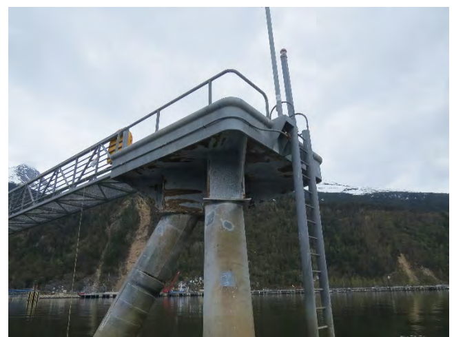
Photo 52- Dolphin addition (6 of 6)
