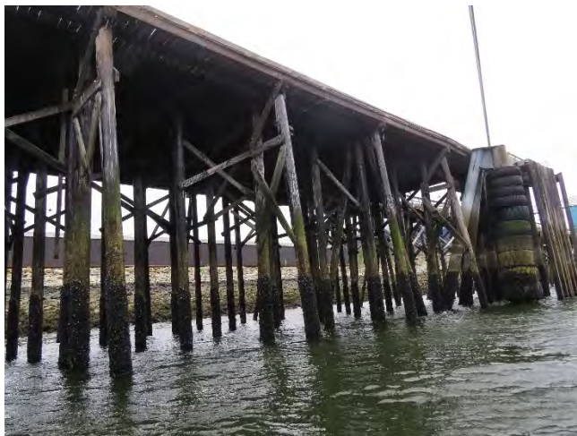
Photo 17- North timber platform (1 of 4)
