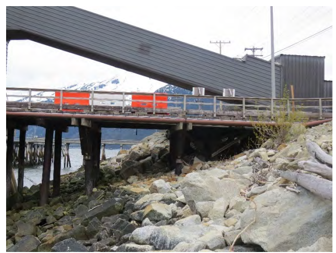
Photo 31- Ore ship loader and timber approach (3 of 6)
