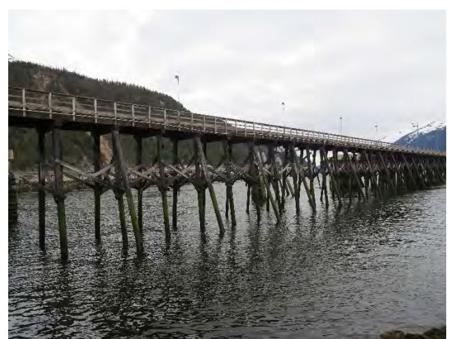
Photo 24- North timber platform (4 of 7)
