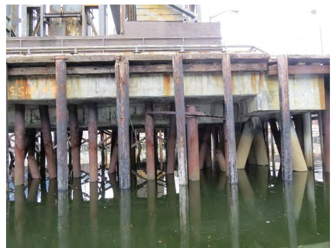
Photo 10- Ore ship loader platform (3 of 3)
