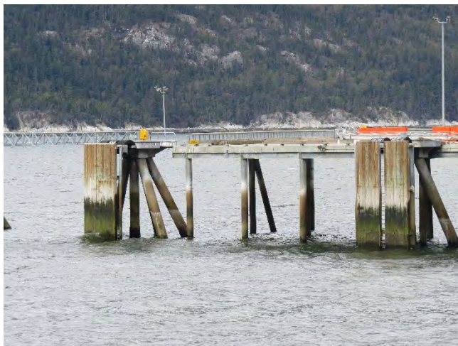
Photo 3- Concrete platform, galv steel with concrete deck (1 of 2)
