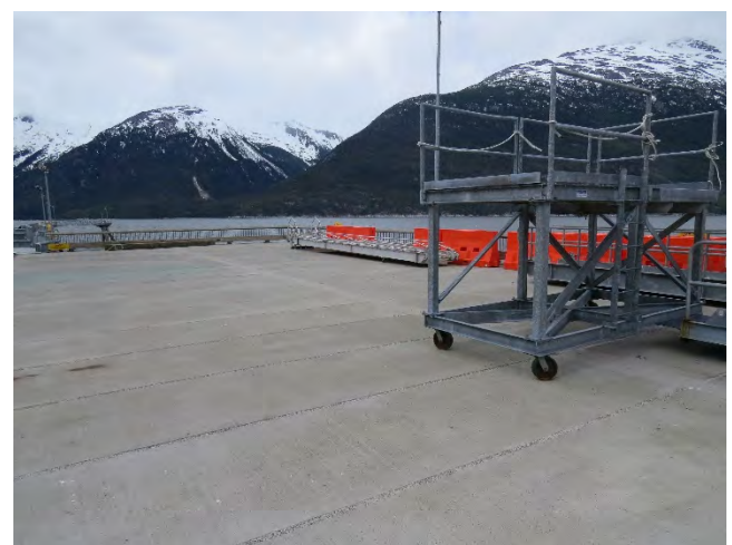
Photo 46- Concrete platform deck (4 of 4)
