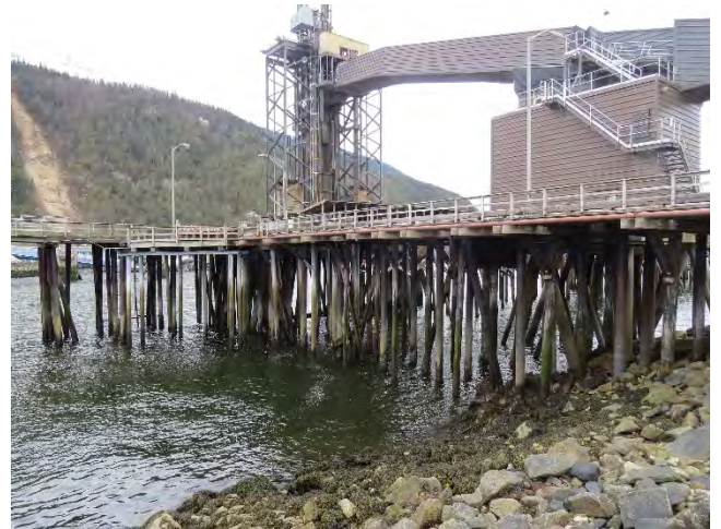
Photo 29- Ore ship loader and timber approach, (1 of 6)
