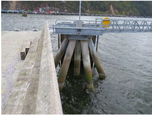
Photo 47- Dolphin addition (1 of 6)
