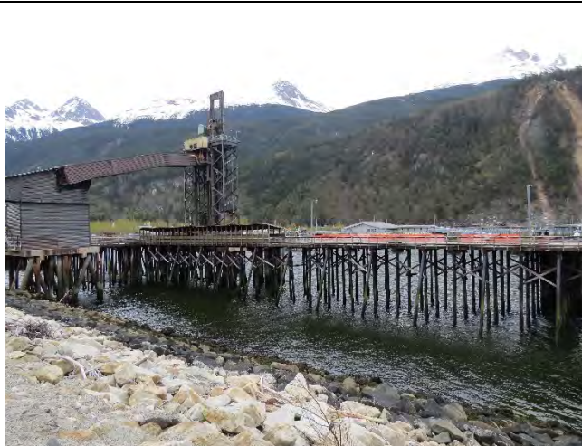
Photo 34- Ore ship loader and timber approach (6 of 6)
