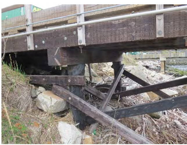
Photo 21- North timber platform, west side (1 of 7)
