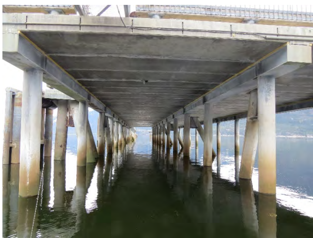
Photo 40- Concrete platform (3 of 4)
