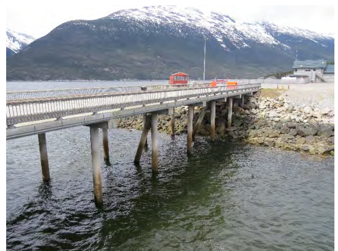
Photo 41- Concrete platform (4 of 4)
