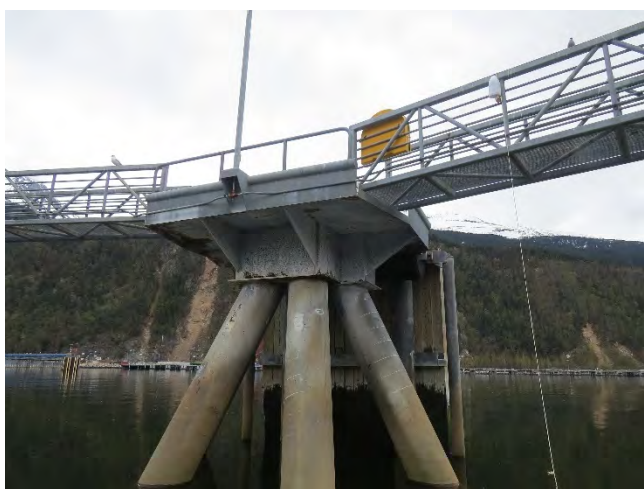
Photo 51- Dolphin addition (5 of 6)
