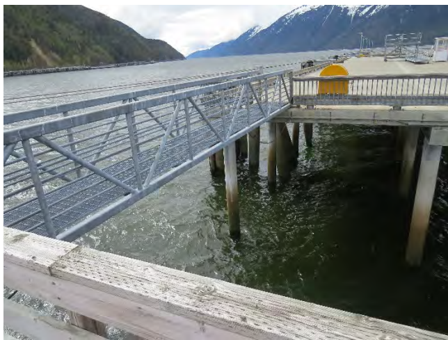
Photo 38- Concrete platform, north elevation (1 of 4)
