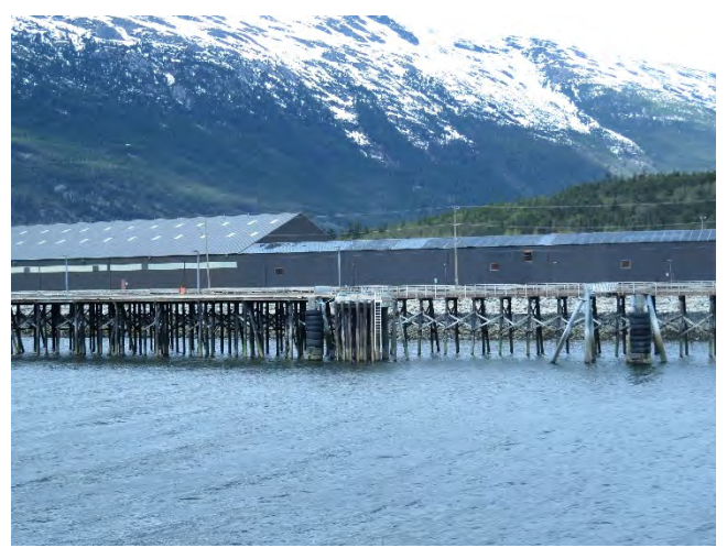
Photo 14- North timber platform (2 of 3)
