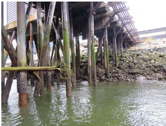
Photo 84 - Alternating steel and wood columns
