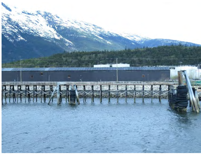
Photo 15- North timber platform (3 of 3)
