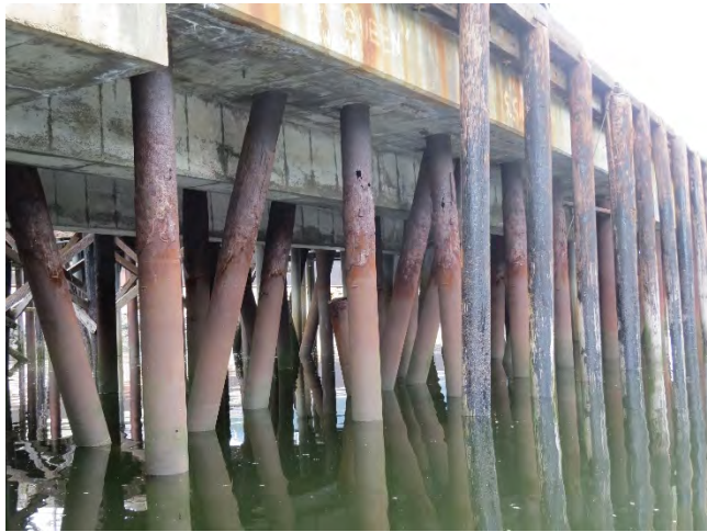
Photo 79 - Old piles left- in-place (1 of 2)
