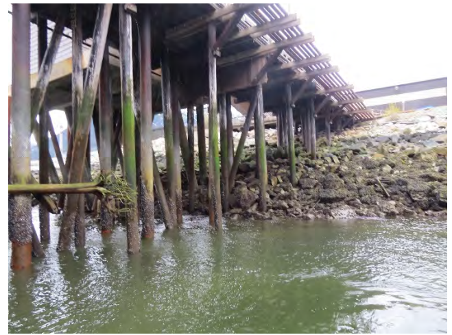
Photo 20- North timber platform (4 of 4)
