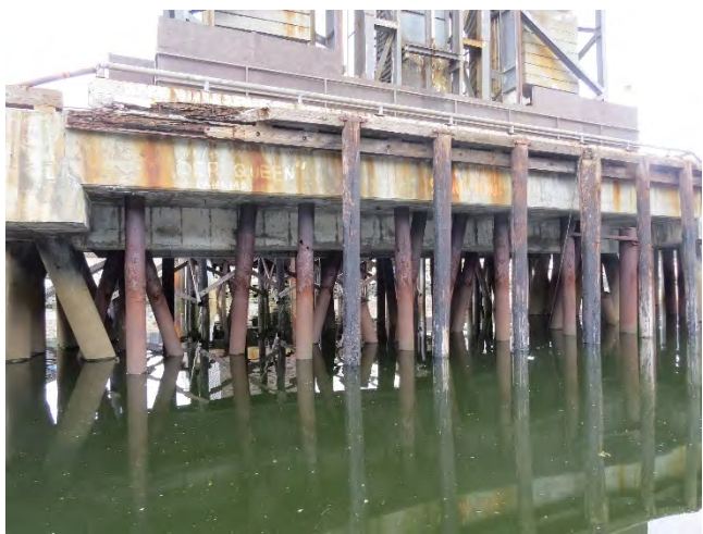
Photo 9- Ore ship loader platform (2 of 3)
