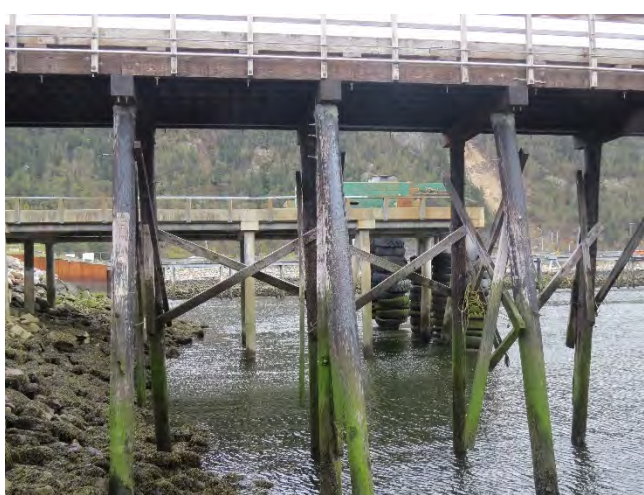
Photo 23- North timber platform (3 of 7)
