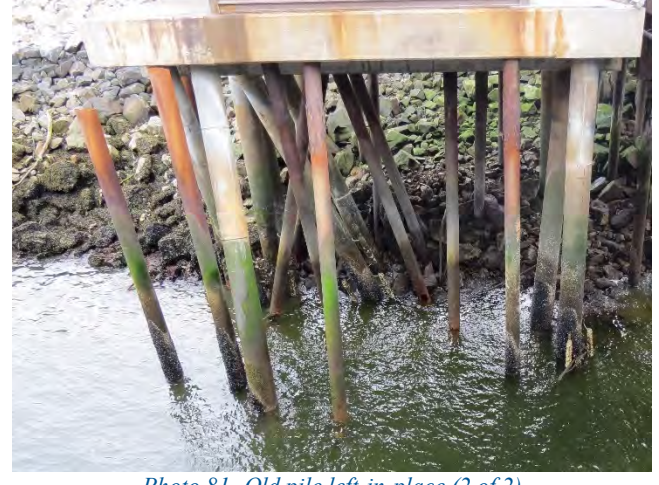
Photo 81- Old pile left-in-place (2 of 2)
