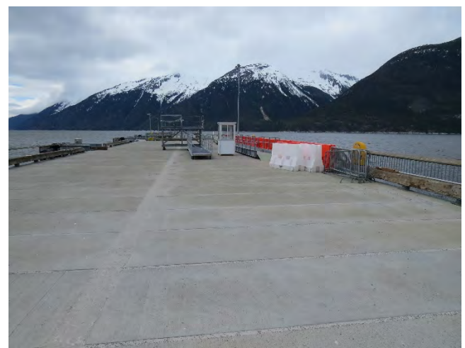
Photo 44- Concrete platform deck (2 of 4)
