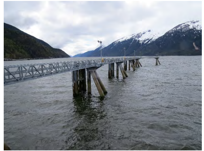
Photo 48- Dolphin addition (2 of 6)
