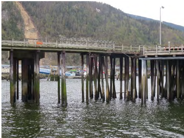
Photo 28- North timber platform (7 of 7)
