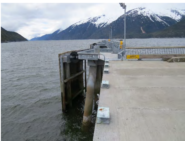
Photo 45- Concrete platform deck (3 of 4)
