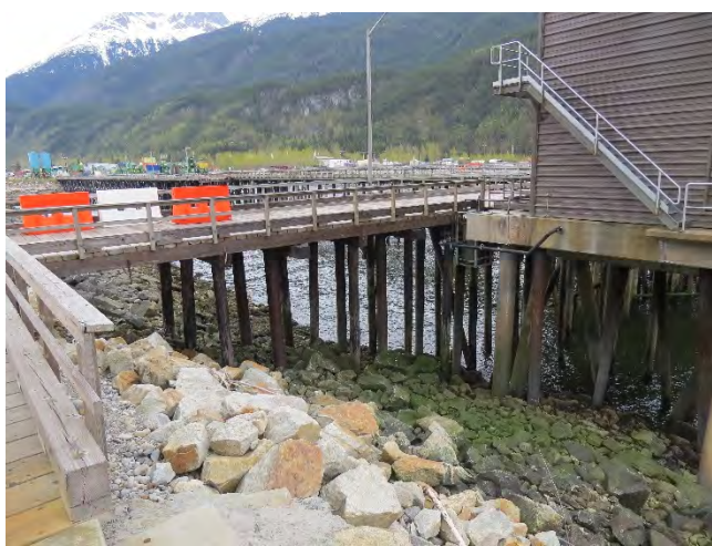
Photo 32- Ore ship loader and timber approach (4 of 6)
