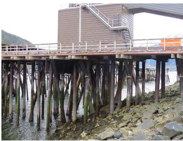
Photo 30- Ore ship loader and timber approach (2 of 6)
