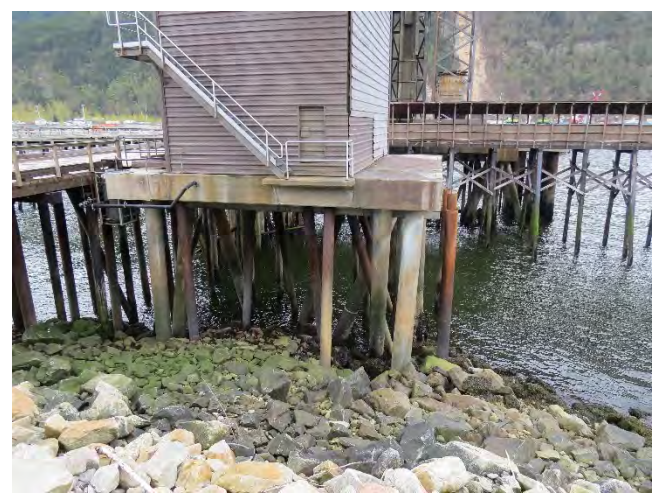
Photo 33- Ore ship loader and timber approach (5 of 6)
