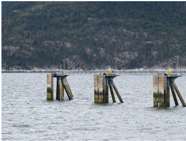
Photo 1- Dolphin addition, galv. steel (1 of 2)
