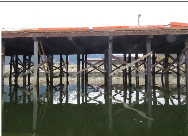
Photo 5- South timber platform (1 of 2)
