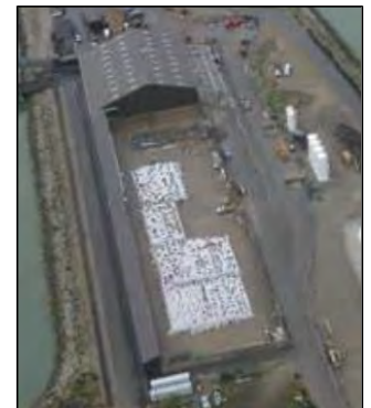
concrete pad staging area
