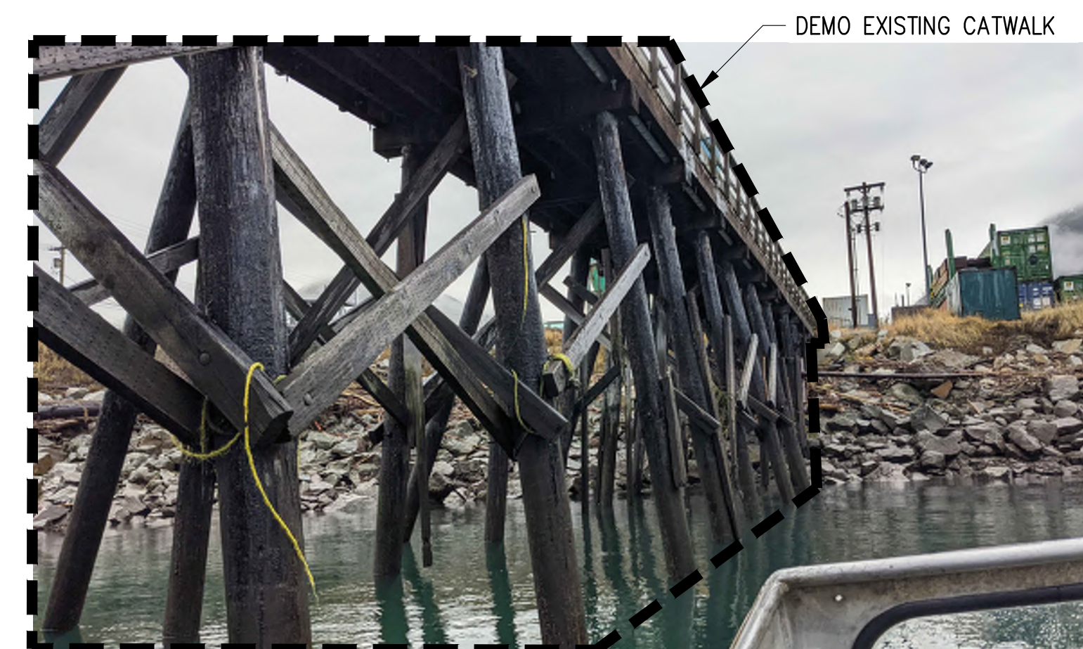
P18 PHOTO EXISTING STRUCTURE ADJACENT TO AML DOCK
