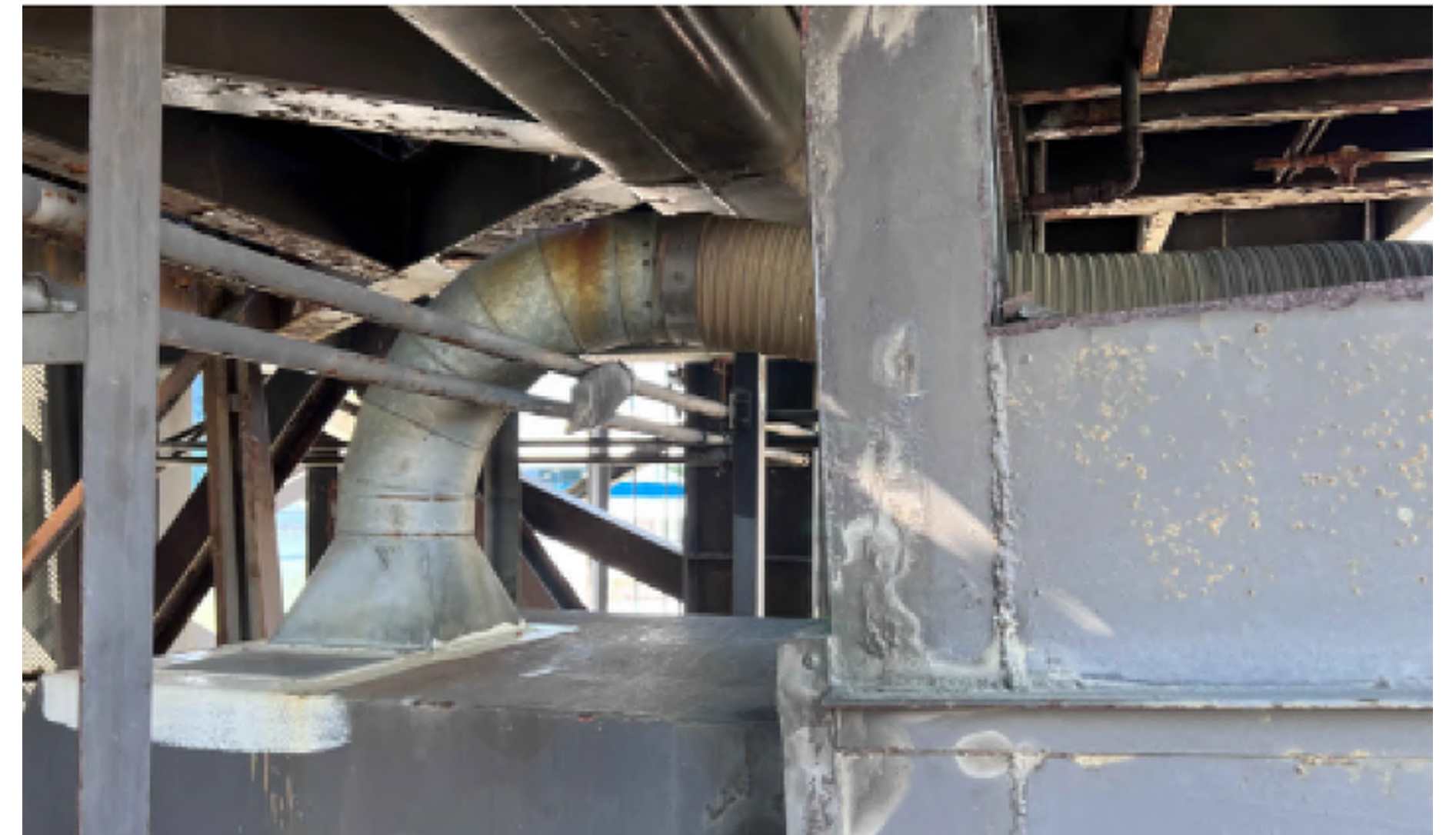
5 D2.10 DEMO CONVEYOR NO. 2 DUST COLLECTION BELOW HYDRAULIC POWER UNIT ROOM
