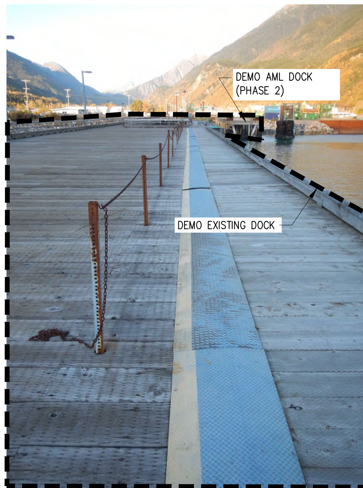
P16 PHOTO EXISTING TIMBER DOCK
