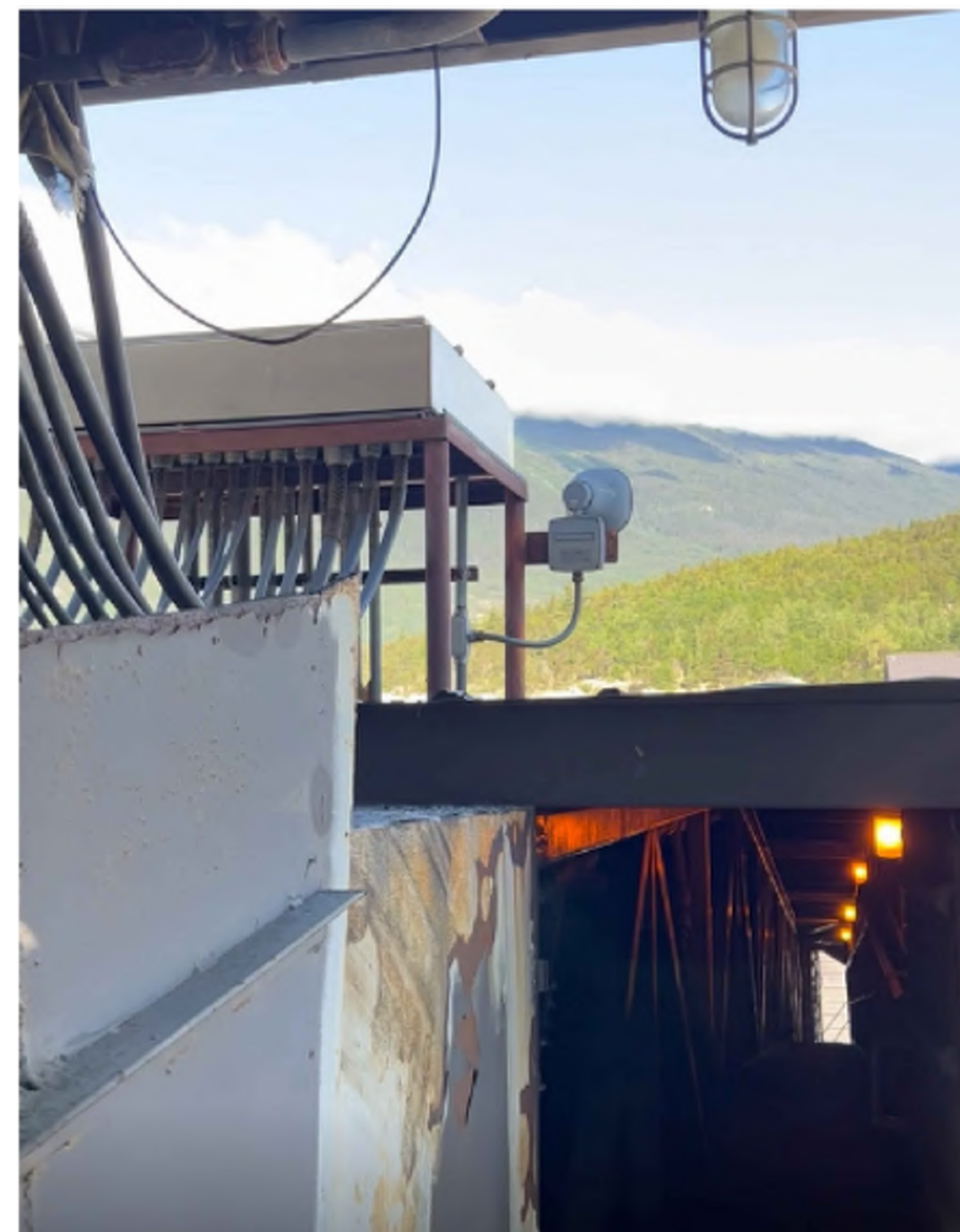
4 D2.10 DEMO CONVEYOR NO. 2 FROM BELOW HYDRAULIC POWER UNIT ROOM
