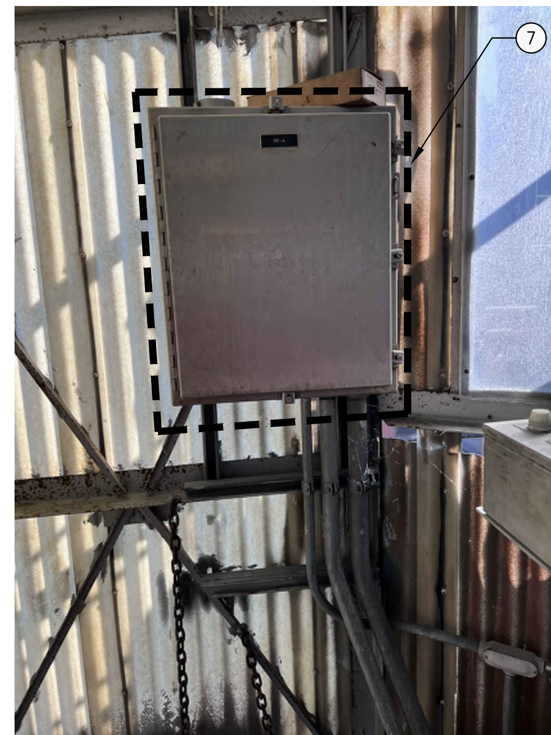
8 D2.20 DEMO SHIP LOADER BOOM CONTROL JUNCTION BOX
