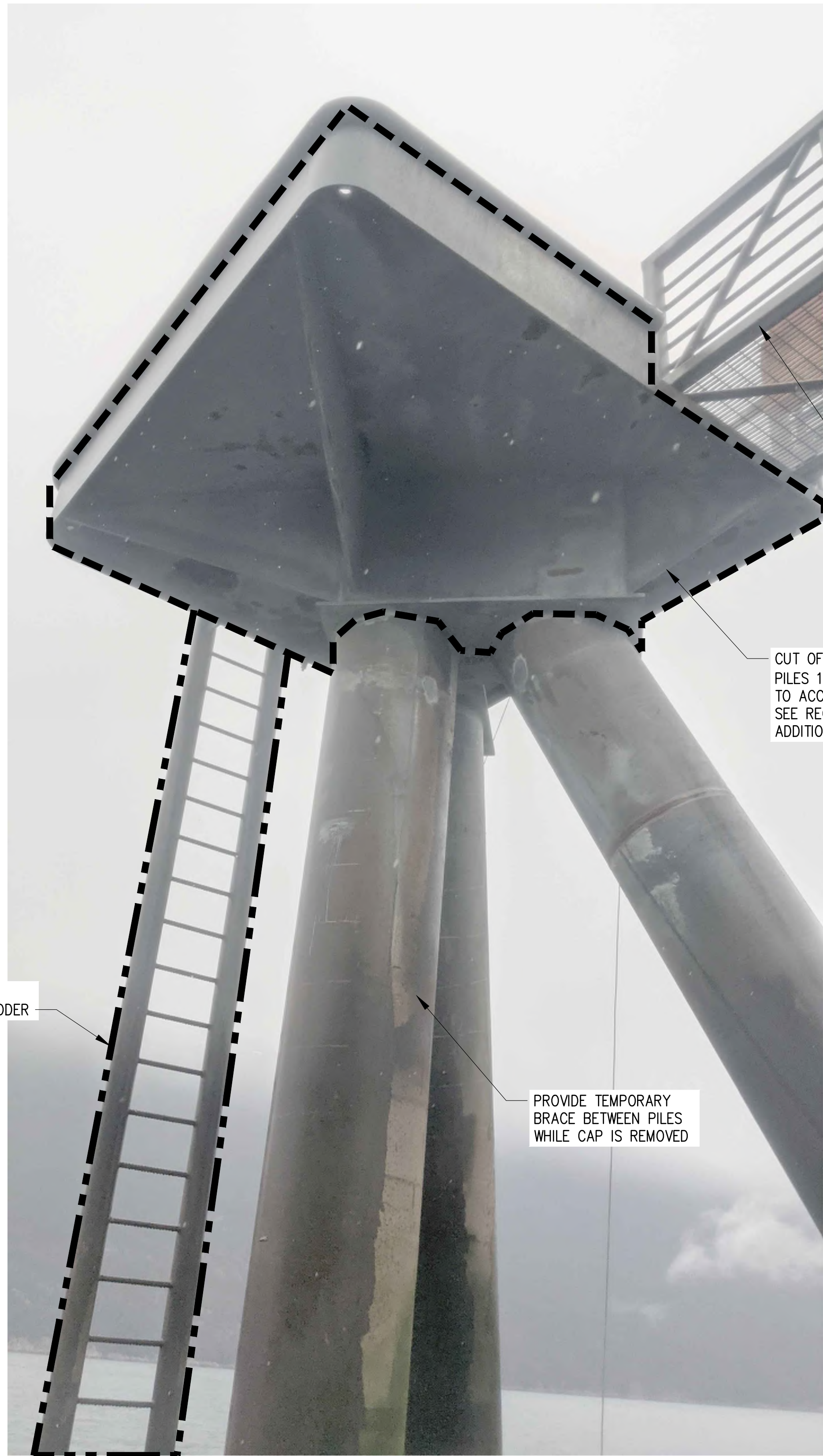
P12 PHOTO EXISTING DOLPHIN A
