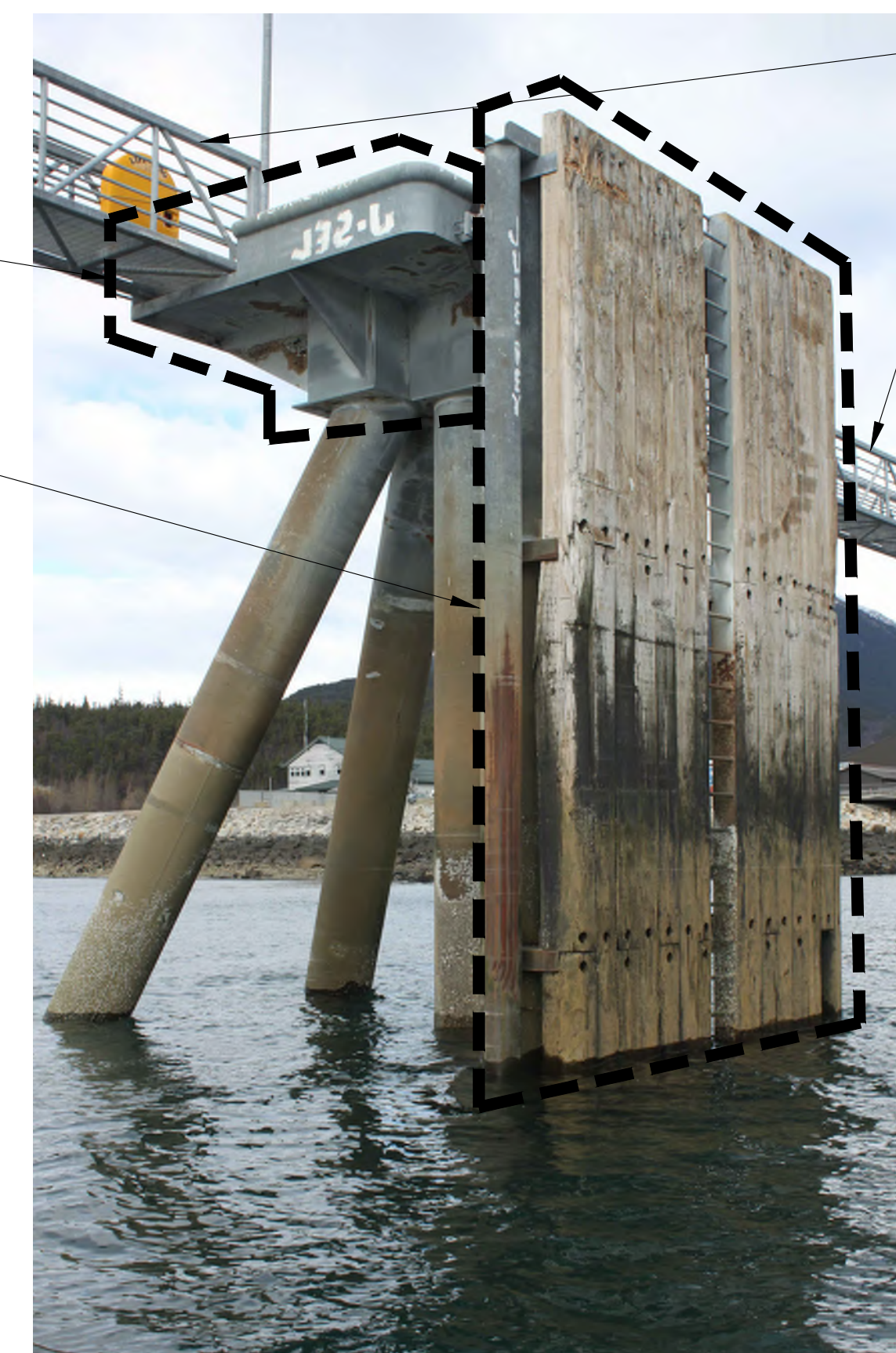
P20 PHOTO EXISTING DOLPHIN B
