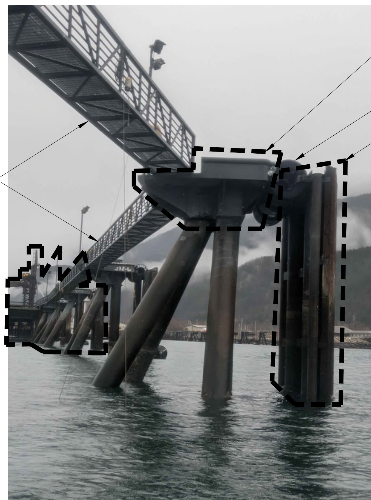
P19 PHOTO EXISTING DOLPHIN B
