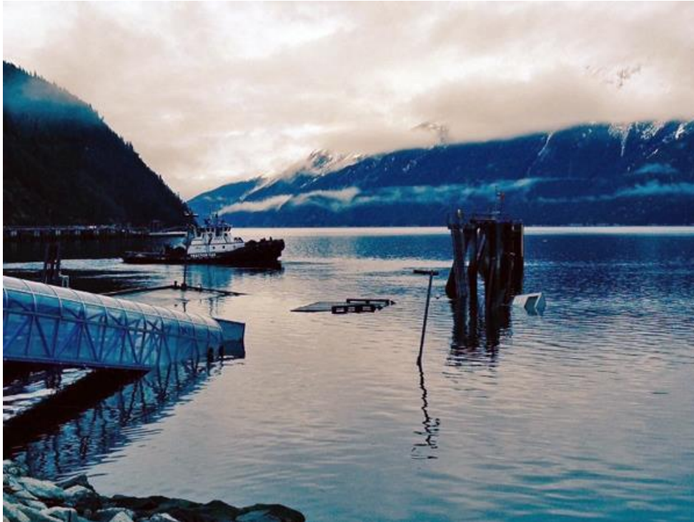
Photo of Skagway Ferry Float after sinking in April 2014
