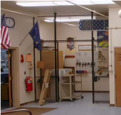
A106 – Metal Screen in Shop
