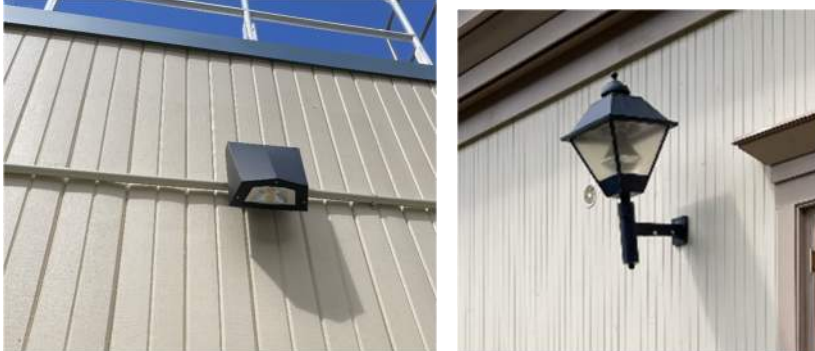
Site Lighting – LED lights on Kitchen Addition (left); wall-mounted lights on original building (right)
