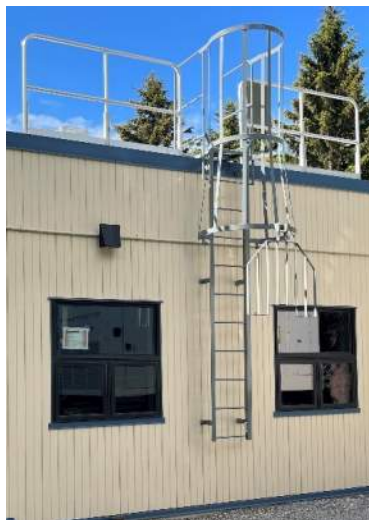
Photo AE45– Roof access ladder at kitchen addition
