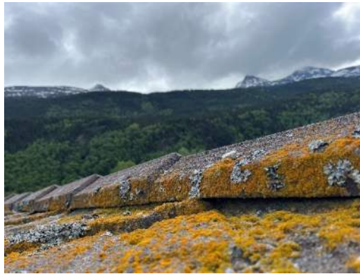
Photo A35 - Reroof 1:12 slope supports growth
