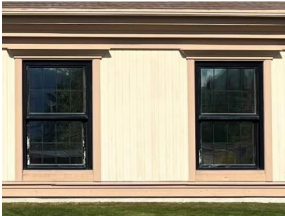
Photo AE06– Orig ext fin cap – window trim, water table
