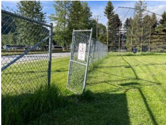
Photo 17 – Out-of-plumb gate
