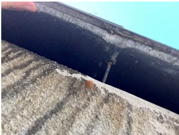
Photo AE44 – Cap flashing at south chase fastening
