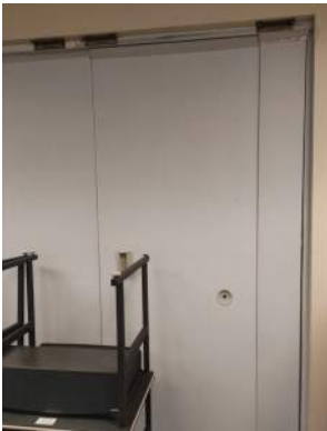
A101 & A102 – Operable partitions in Elementary Classroom wing
