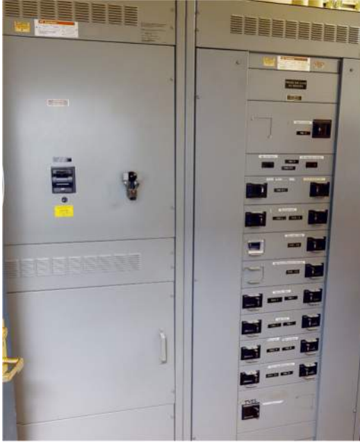
Original Switchgear (left); New Switchgear (right)
