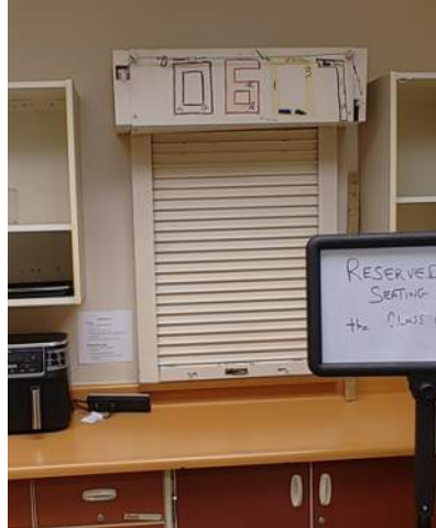
A114 & A115 – Overhead Coiling Counter Doors at Home Ec 33 and Student Store 10.
