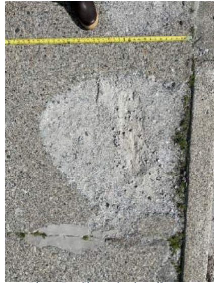
Photo 7 – Chipped sidewalk
