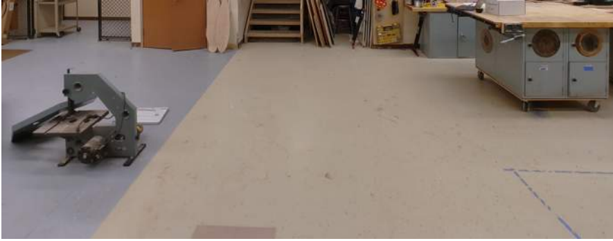
AI24 – Painted Concrete Floor
