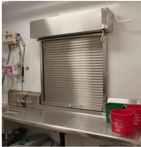
A112 & A113 – Overhead Coiling Counter Doors at Office 1 and Kitchen 30
