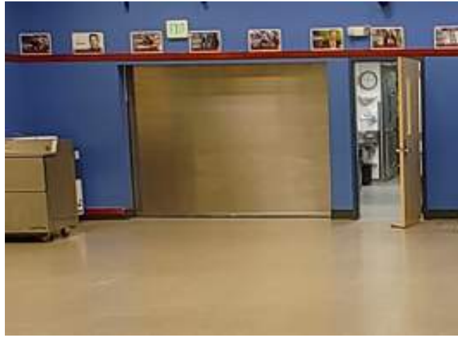
A110 & A111 – Overhead Coiling Door at Shop Mezzanine and Kitchen 30
