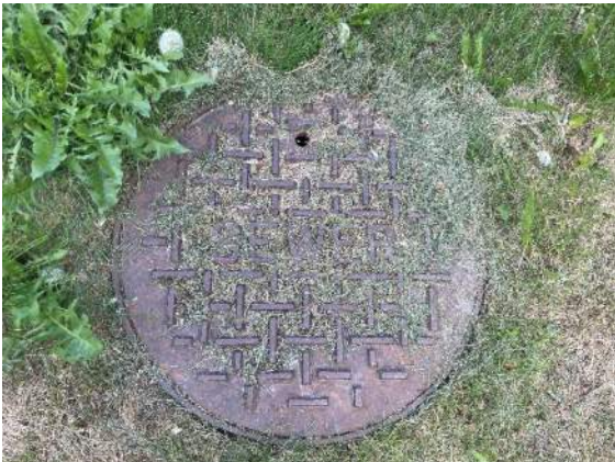
Photo 35 – Sanitary sewer manhole
