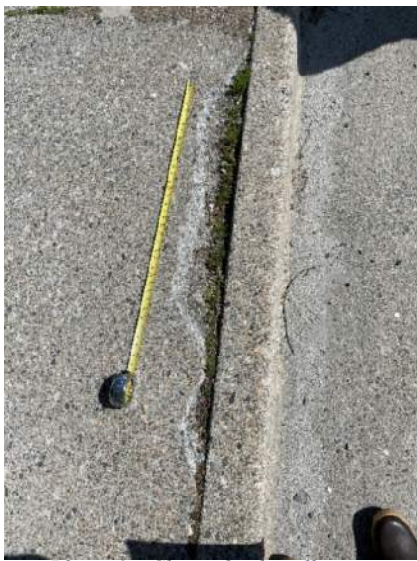
Photo 6 – Chipped sidewalk
