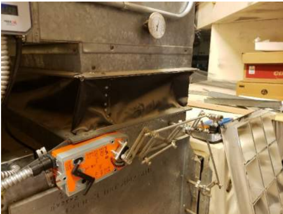
Mixing Box Control Dampers
