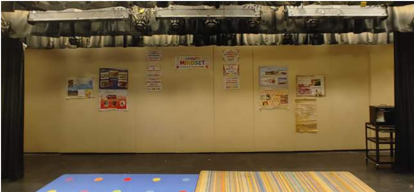
AI04 – Operable partitions in Elementary Classroom wing
