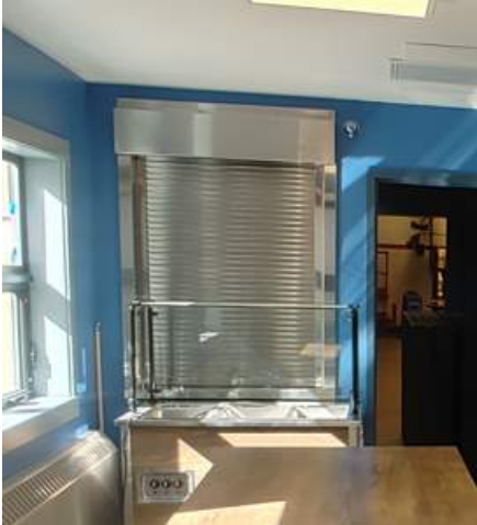
A114 & A115 – Overhead Coiling Counter Doors at Home Ec 33 and Student Store 10.
