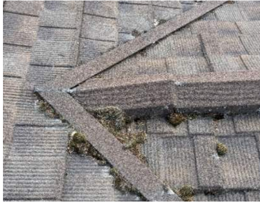
Photo A29 - Reroof 3:12 slope, ridge and valley support growth
