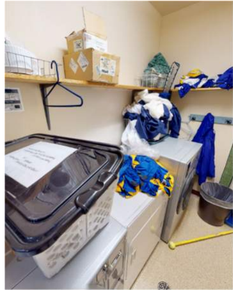
Laundry Room Dryers
