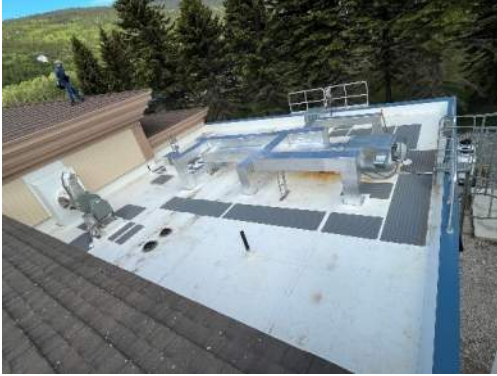
Photo AE41 – Flat roof at kitchen addition
