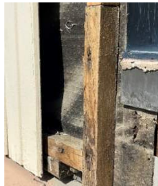
Photo AE02– Orig wood cladding assembly, typ
