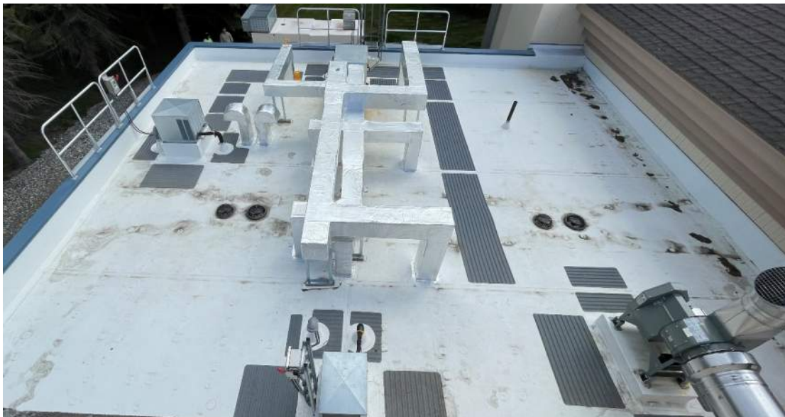
Photo 47 — Flat roof above kitchen.
