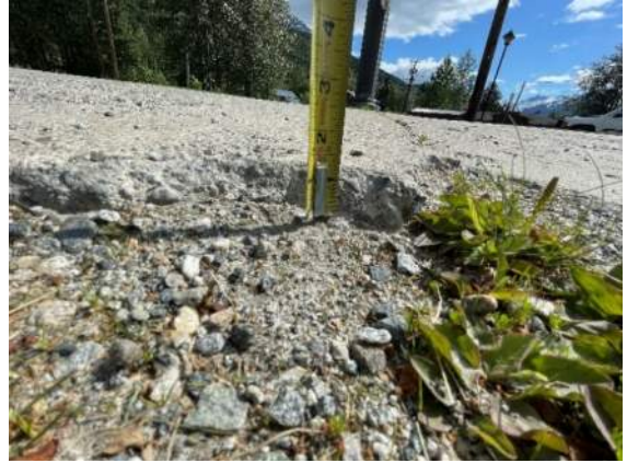
Photo 5 – Chipped sidewalk
