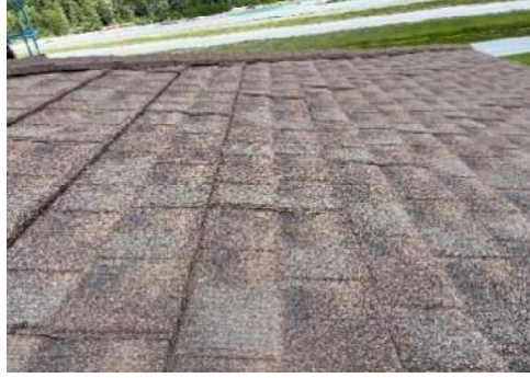
Photo AE27– Reroof 3:12 slope, open edge joints
