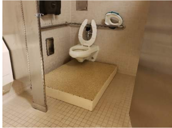
Wood Platform (Girls Restroom 305)
