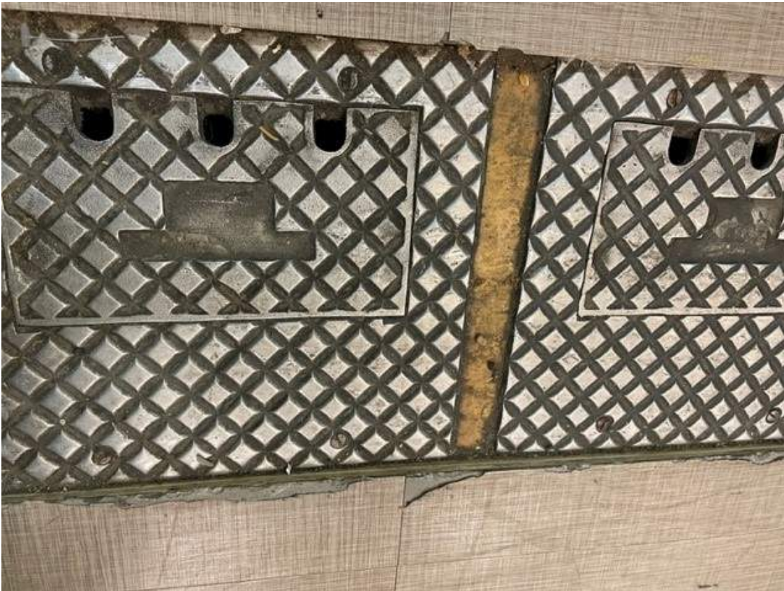
AI24a – Multi-Purpose Room – Vinyl Tile installed over Original Floor
