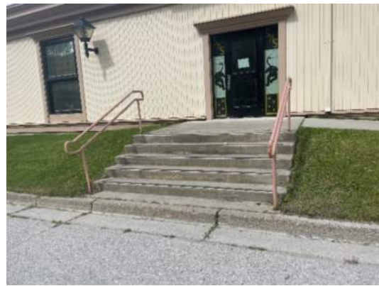
Photo 11 – Exterior door stairs and handrails
