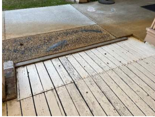
Photo AE25– Orig wood deck at entry
