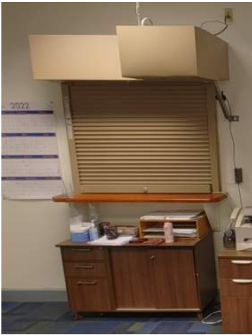
A112 & A113 – Overhead Coiling Counter Doors at Office 1 and Kitchen 30
