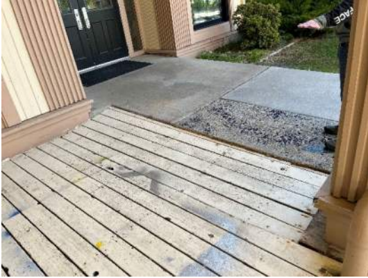
Photo AE24– Orig wood deck at entry
