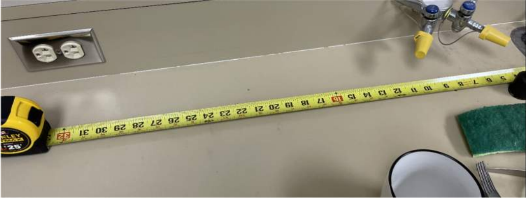
Receptacle near sink above countertop
