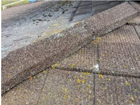
Photo A30 - Reroof 3:12 slope, exp fasteners
