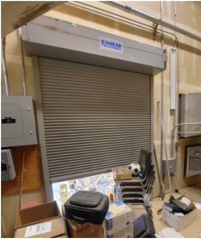
A110 & A111 – Overhead Coiling Door at Shop Mezzanine and Kitchen 30
