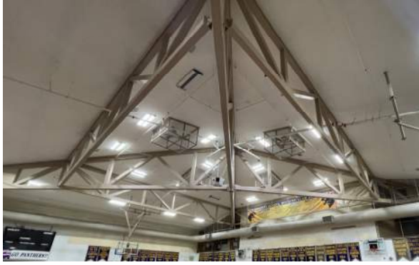
Photo 45 — Tube steel trusses supporting gym roof.
