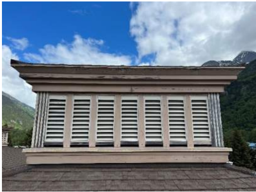
Photo A34 - Reroof 1:12 slope at north cupolas
