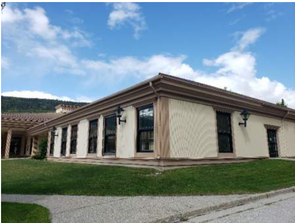
Gutters & Sloped Roofing
