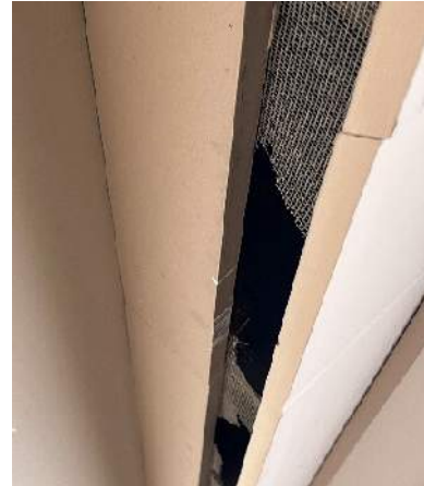
Photo AE11 – Orig vented soffit, typ
