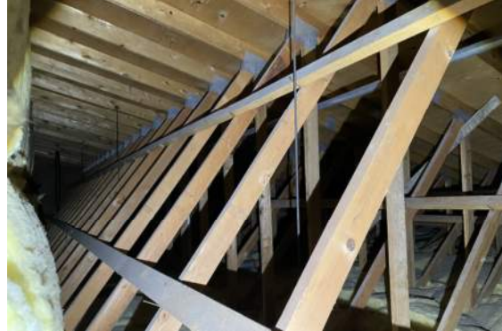
Photo 46 — Pre-engineered wood trusses
