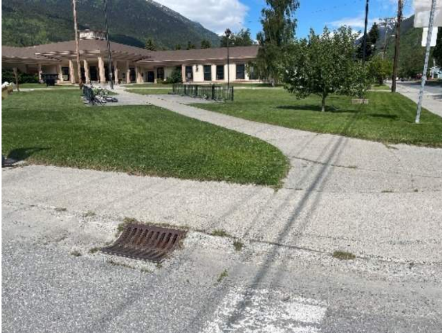
Photo 37 – Storm drain curb inlet along Fifteenth Street
