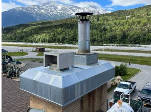
Photo AE43 – Cap flashing at south chase
