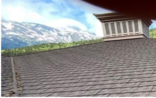
Photo AE26– Reroof 3:12 slope, typ
