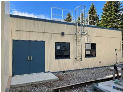
Photo AE03– New wood cladding at kitchen add
