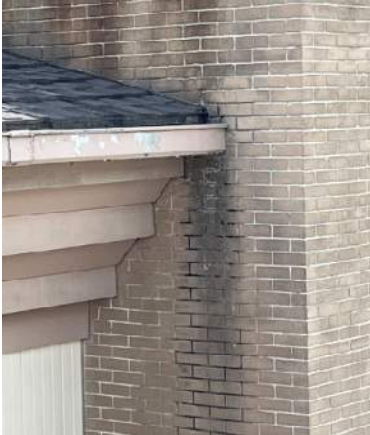
Photo AE39 – Example limited gutter Photo AE40 – Built in gutters use internal downspouts
