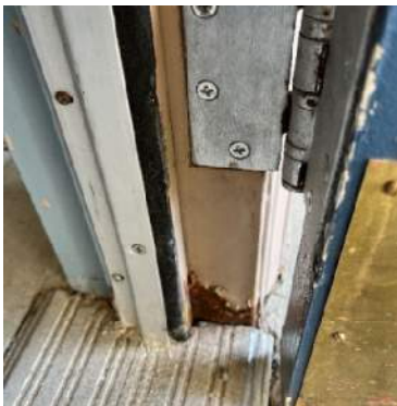
Photo AE19– Door E01, jamb at threshold
