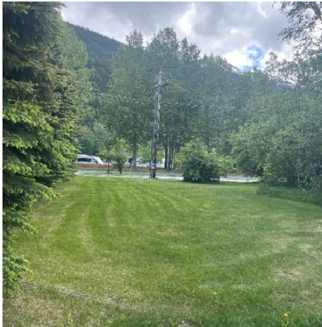
Photo 38 Low spot near generator pad
