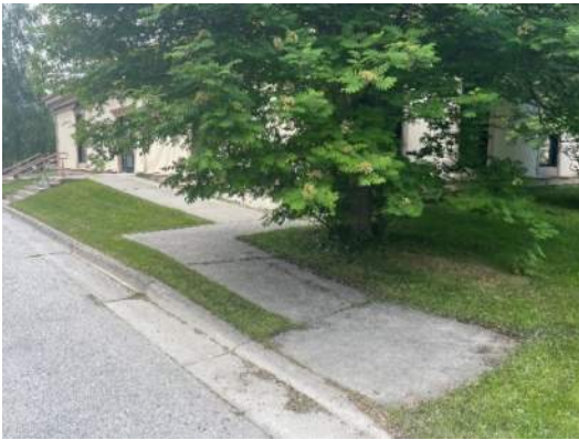
Photo 10 – Ramp from exterior door
