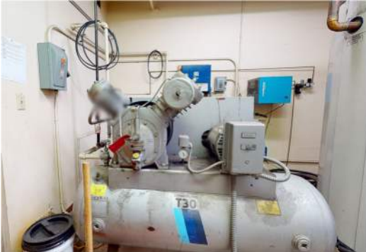
Left to Right: Disconnects blocked by tanks, Disconnects blocked by pumps
