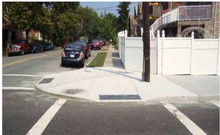
Two examples of corner ‘bulb outs’ and integrated crosswalks, which extend the sidewalk into the street, shortening the distance a pedestrian has to walk, improving line of sight for both drivers and pedestrians, and slowing auto traffic.
