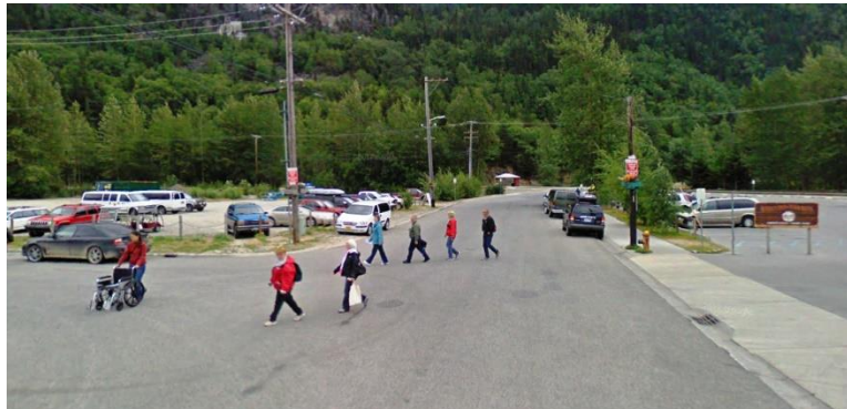
Uncontrolled crossing at intersection of Spring Street and 2 nd Avenue, looking east toward Railroad Tracks. Sidewalk on north (left) side is needed, crosswalk is needed. Photo: Google Earth Street view
